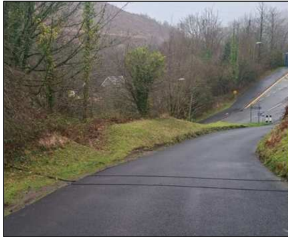
FIGURE 2.10: ATC 1 IN PLACE
