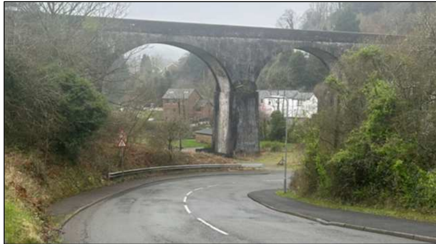
FIGURE 2.6: QUEEN STREET (SOUTH OF OAKWOOD AVENUE)
