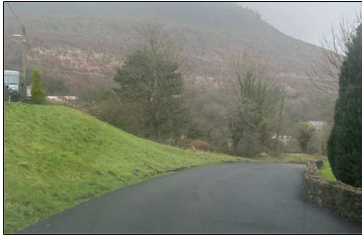
FIGURE 2.3: OAKWOOD AVENUE (NEAR B4287)
