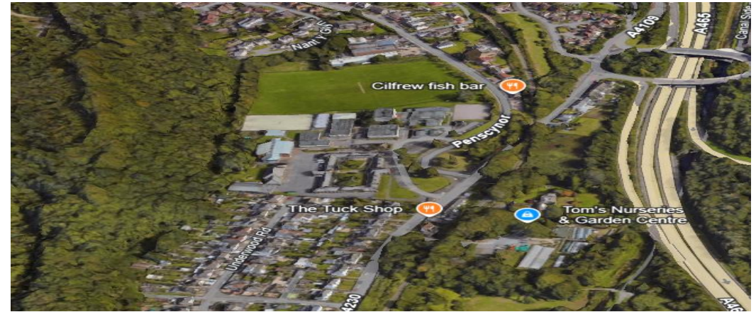
Fig.1.10 – Aerial View of Site in Context with Surrounding Townscape
