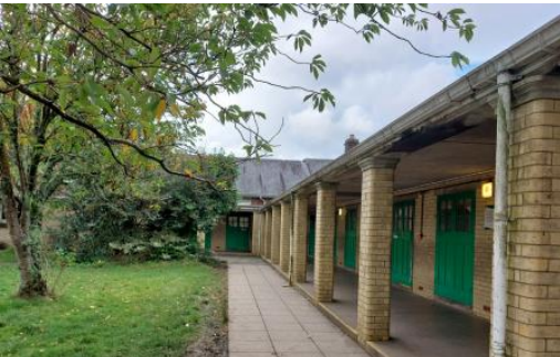
Fig.1.8 – Example of existing building & School areas
