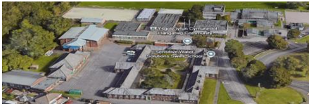
Fig.5.1 – Existing school demolished in Phase 2
