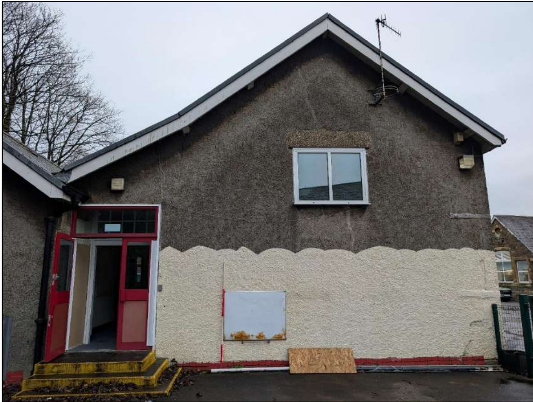
Plate 5. West facing elevation, view to the east.
