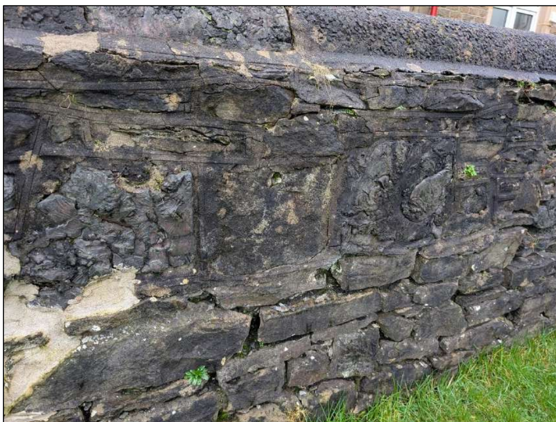
Plate 48. Eastern side of boundary wall showing the slag used within construction, view to the north-west.
