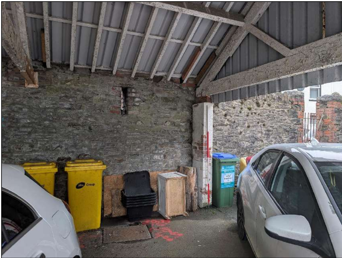
Plate 51. Brick supports within the interior of the shed, view to the north-west.
