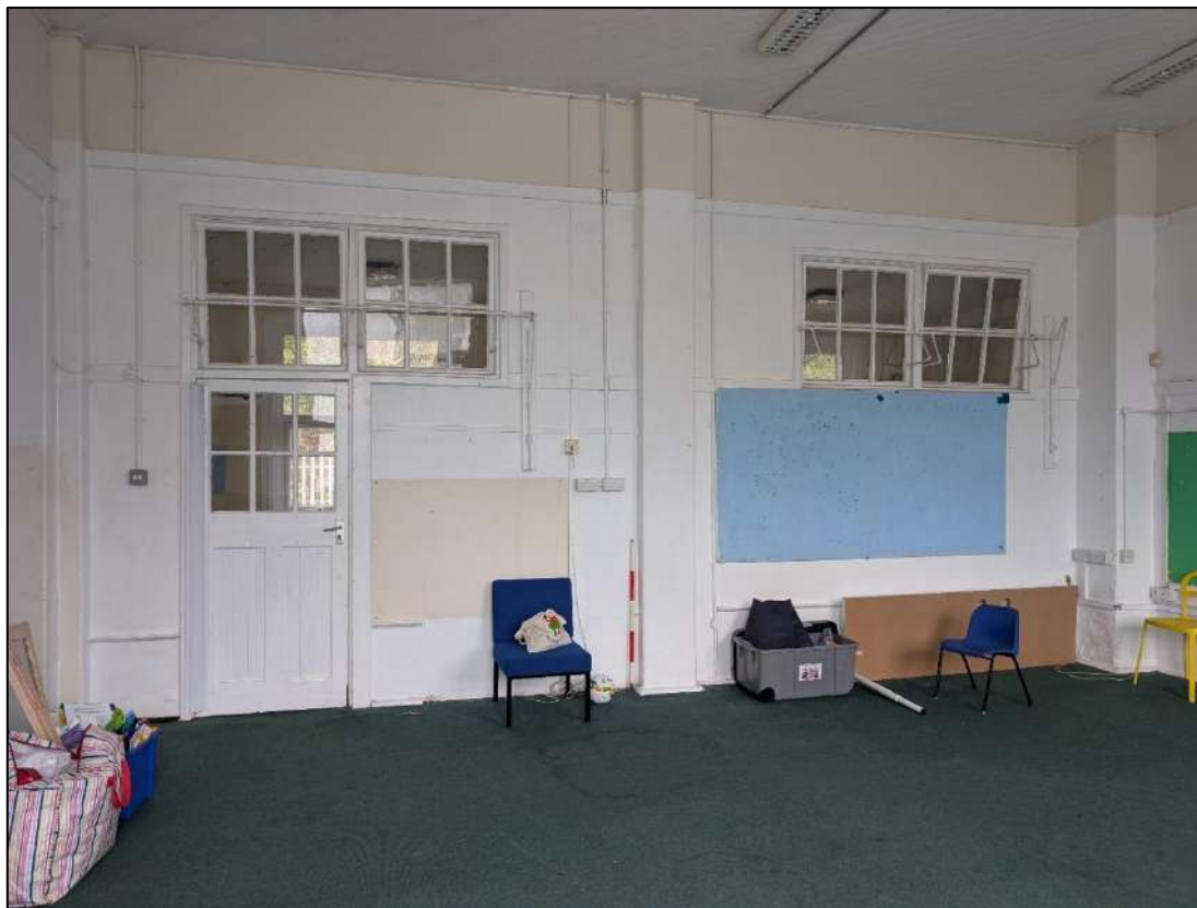
Plate 19. Northern wall of classroom, view to the north-east.
