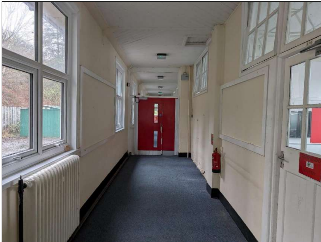
Plate 26. Central corridor, view to the east.
