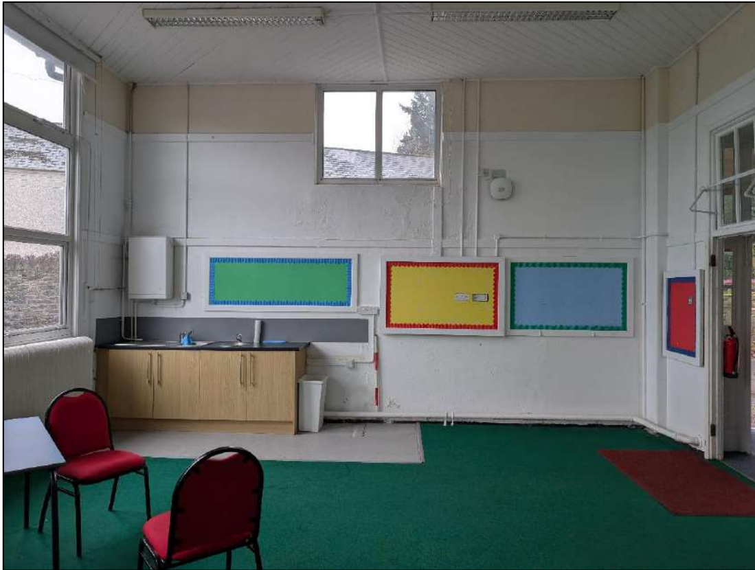
Plate 21. High level window on the western wall, view to the west.
