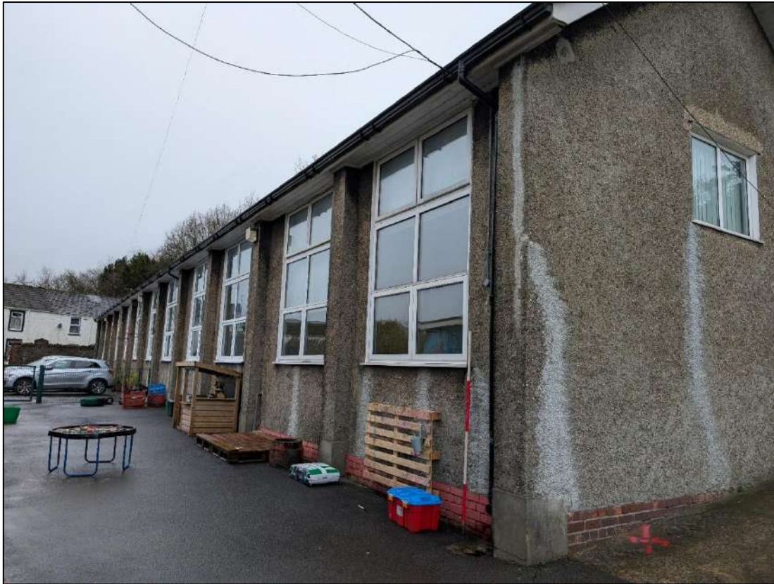
Plate 1. South facing elevation, view to the west-north-west.
