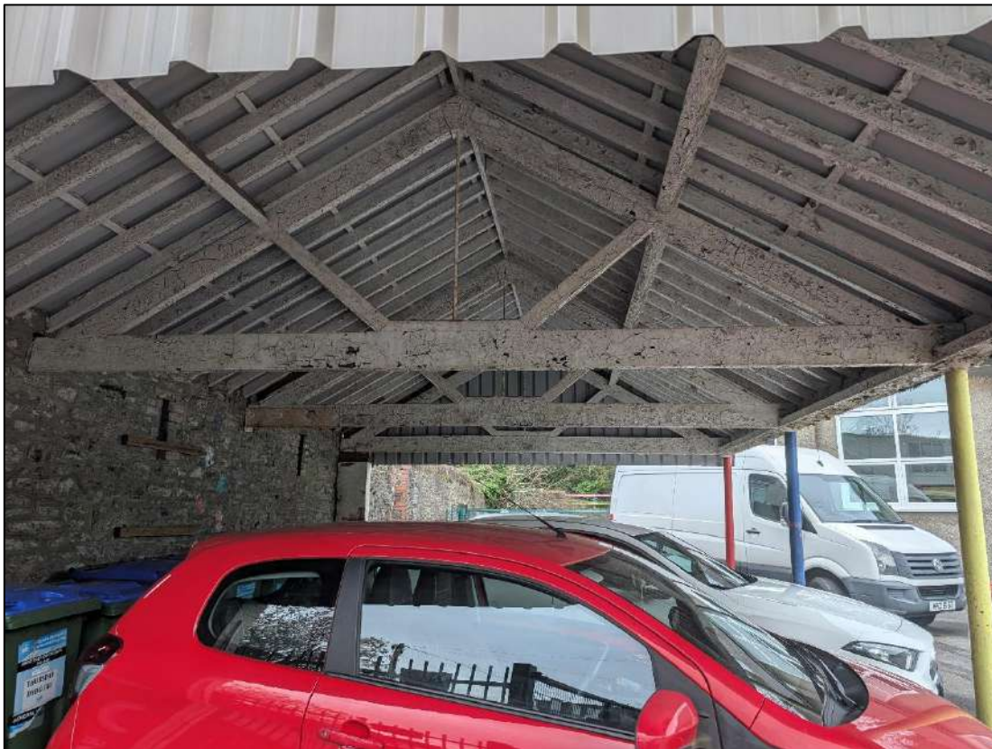
Plate 52. Timber and steel roof trusses within shed, view to the north.
