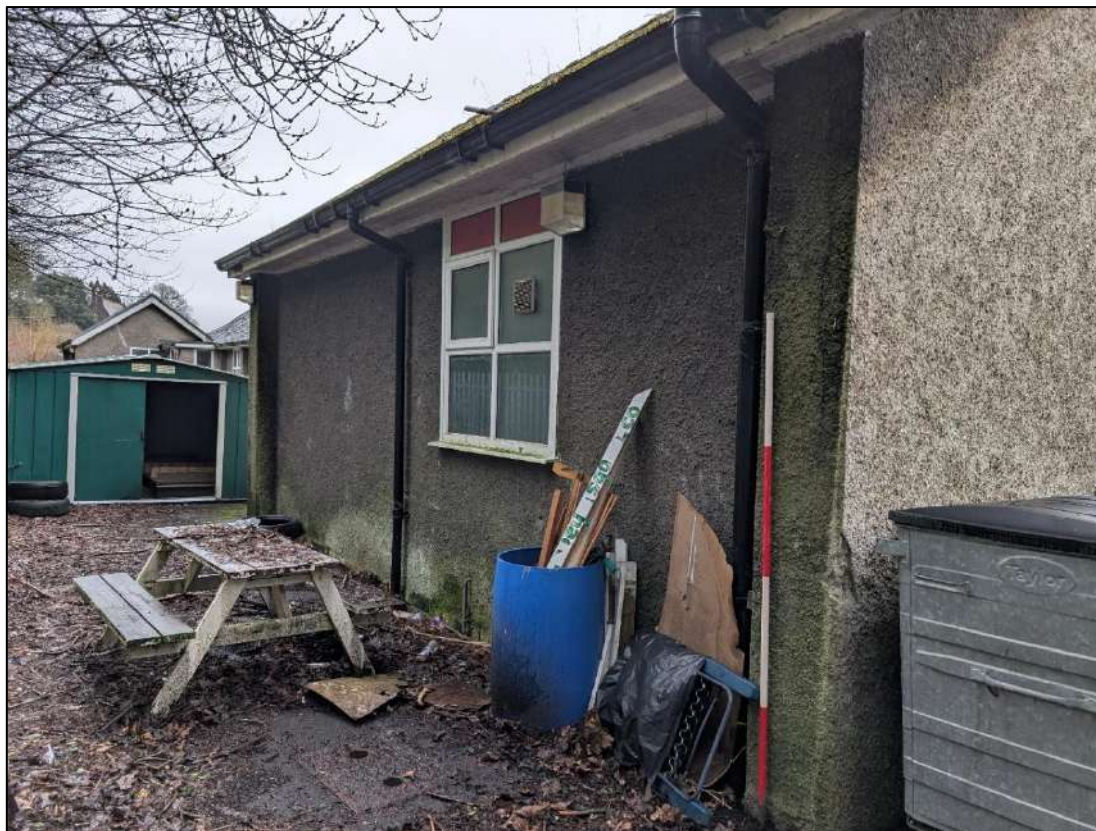
Plate 9. North facing elevation of western range, view to the south-east.
