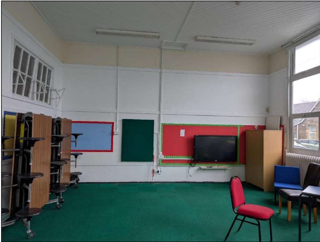
Plate 17. View of the boarded ceiling within classroom, view to the east.
