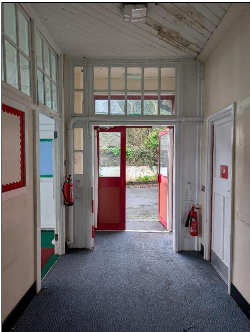
Plate 23. Interior of rear entrance, view to the west.
