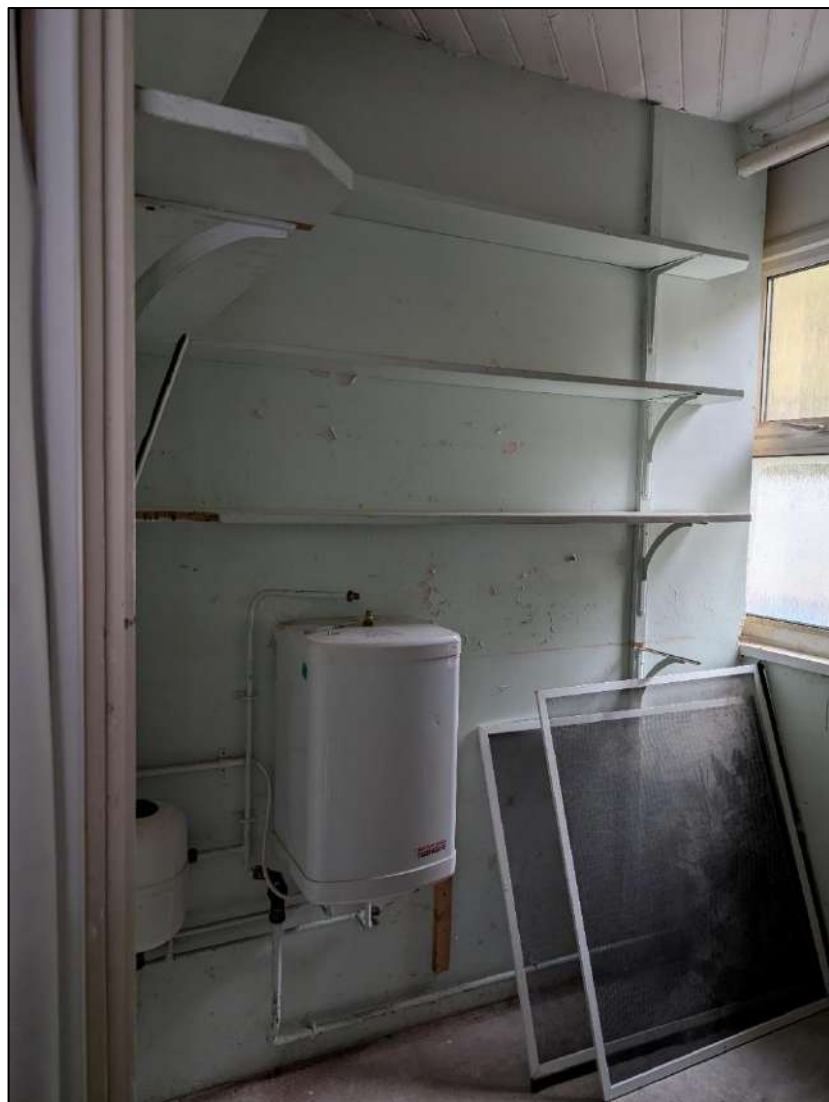
Plate 41. Room 15, view to the north-west.
