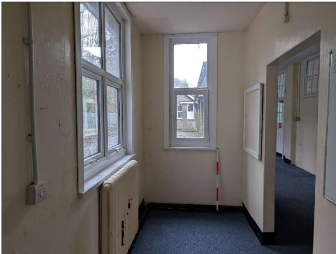
Plate 38. Room 13 view to the east.
