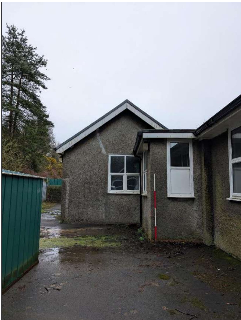
Plate 15. West facing elevation of eastern square extension, view to the east
