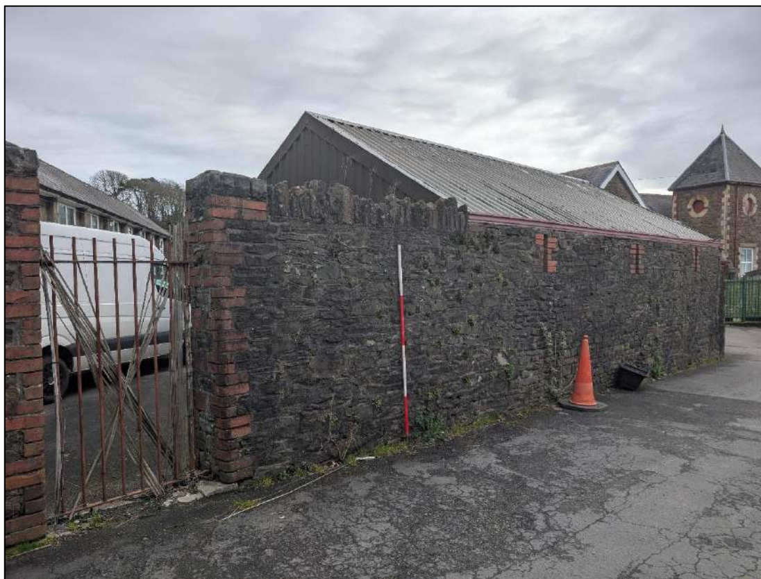
Plate 49. Western elevation of boundary/shed wall, view to the south-east.
