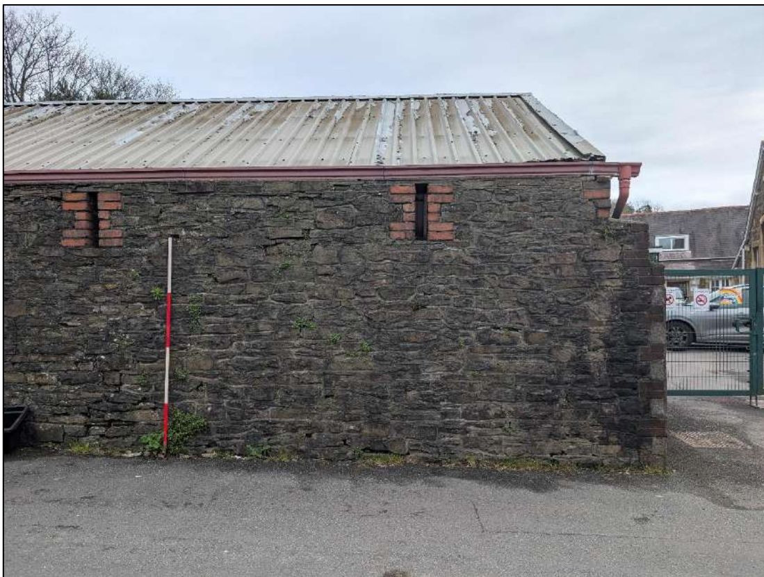
Plate 54. Boundary wall at main entrance, view to the north-east.
