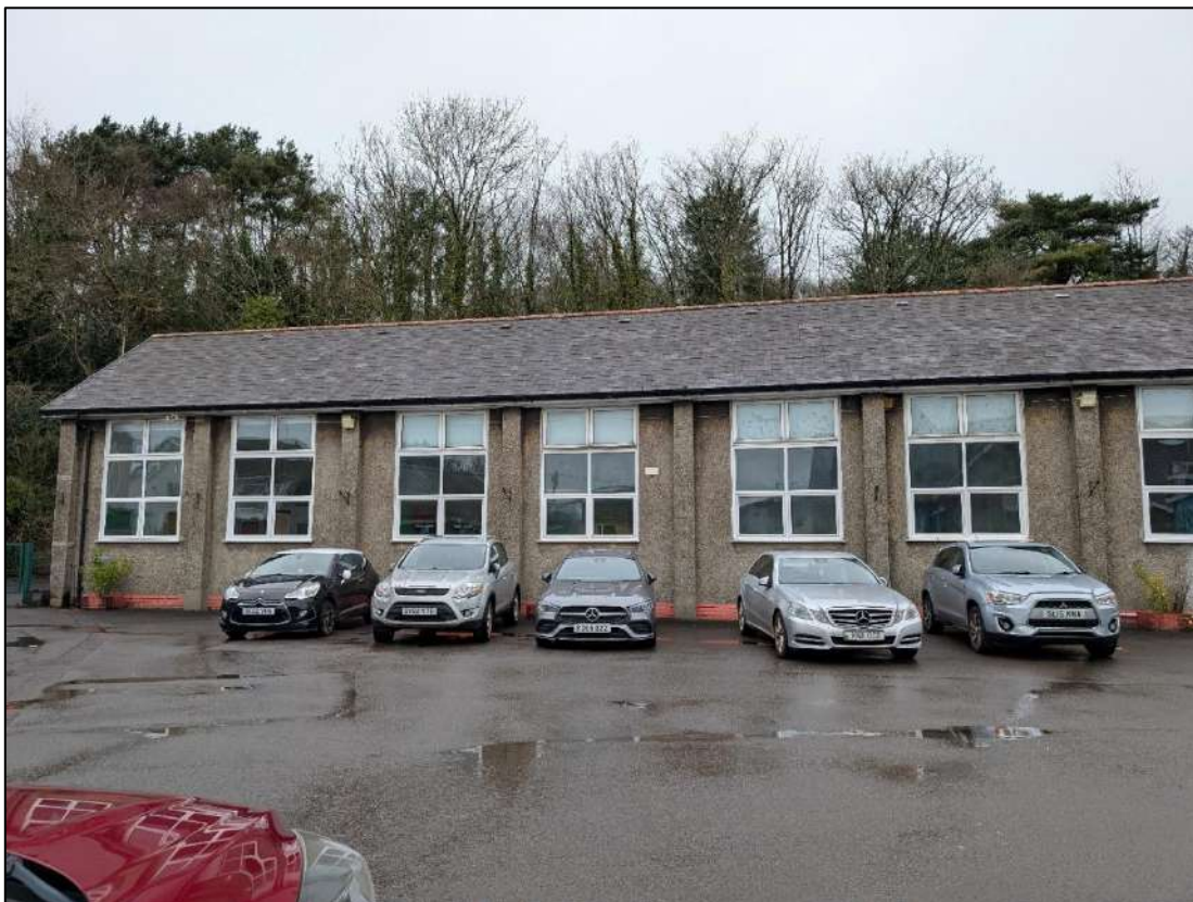
Plate 2. South facing elevation, view to the north.
