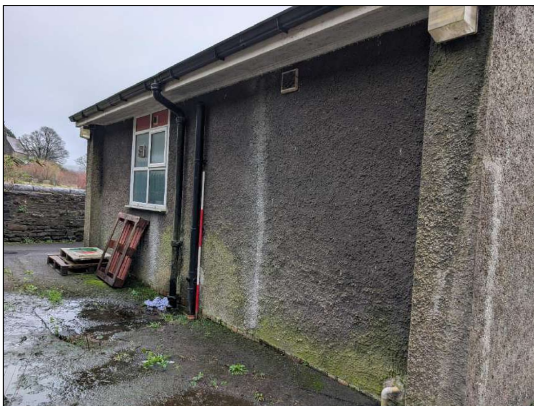
Plate 10. North facing elevation of eastern range, view to the south-east.
