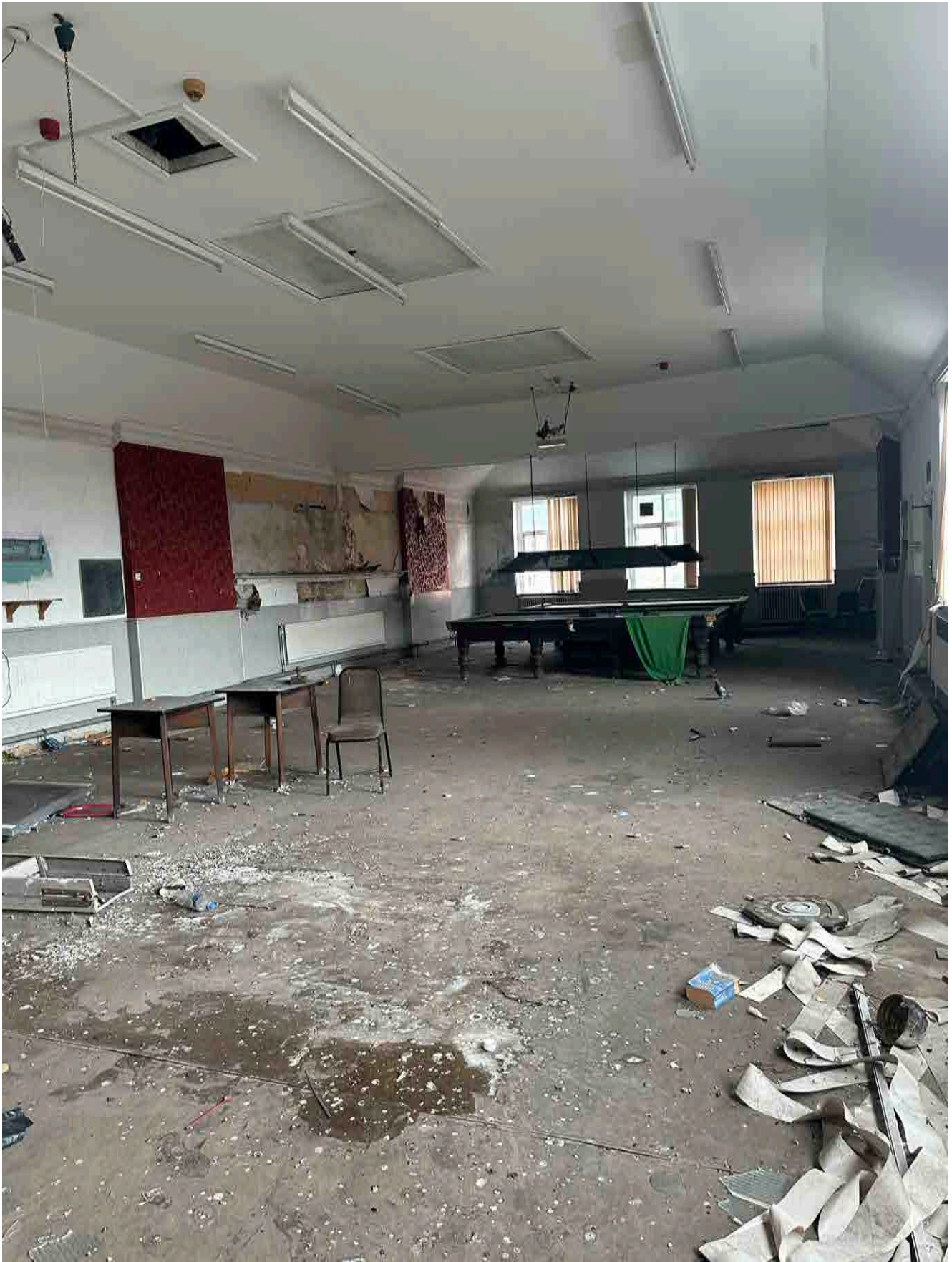
The rear room on the first floor
