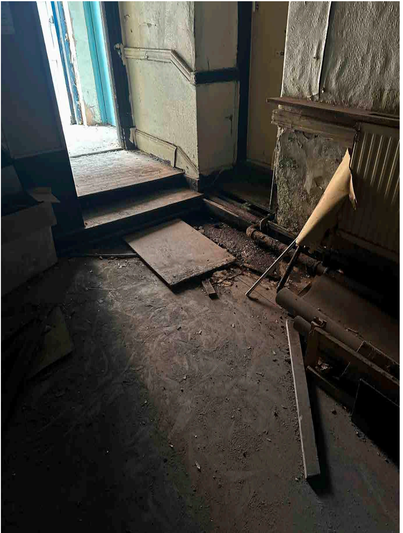
Suspended timber ground floor in the rear section of the building
