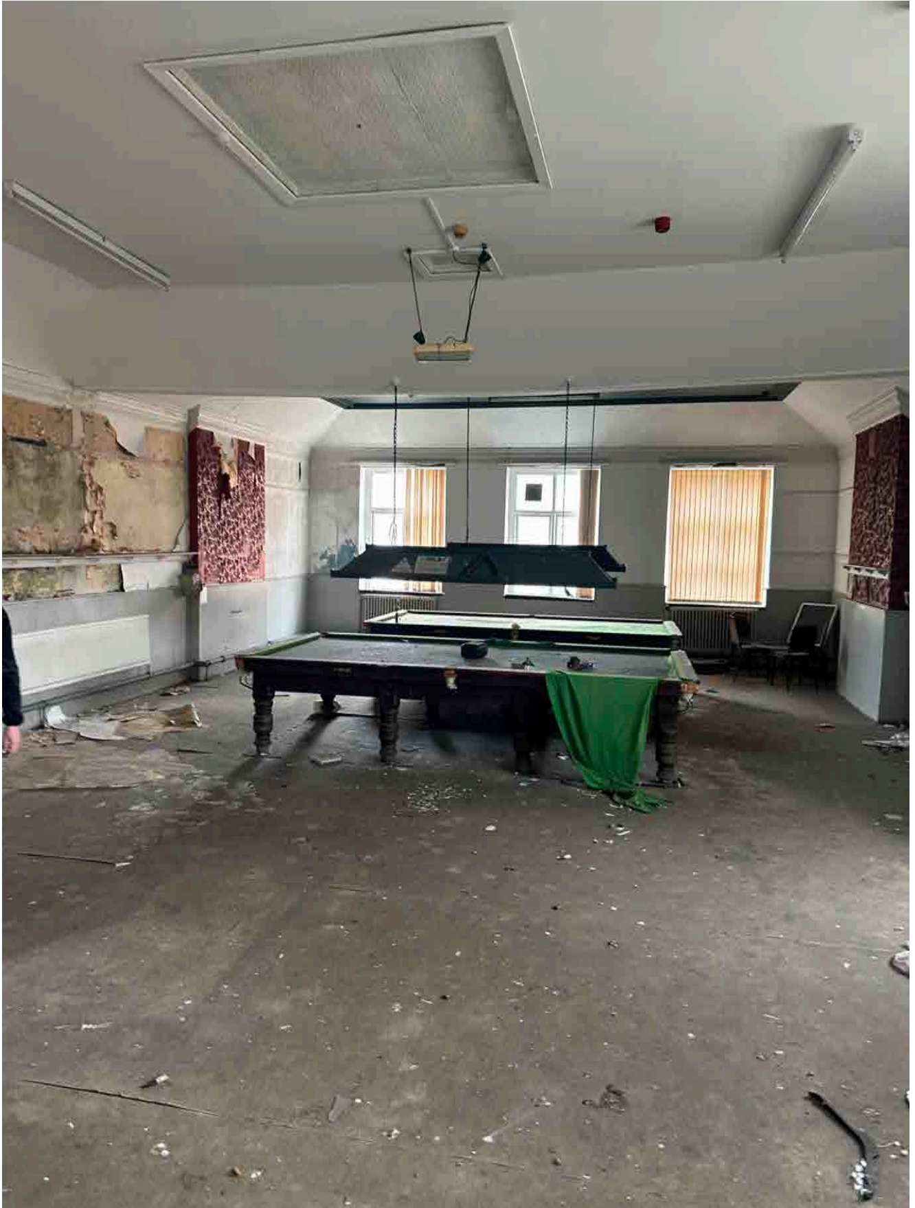
The truss in the rear first floor room shows signs of bowing and should be strengthened
