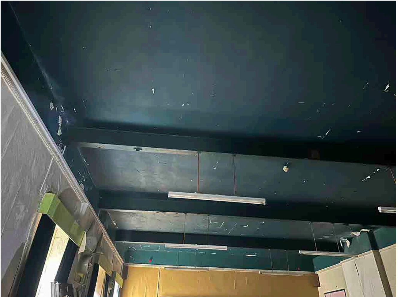
First floor supported by steel beams
