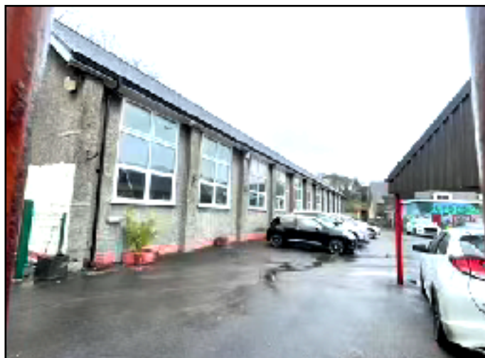
Photo 12. Central hardstanding parking area within school buildings.
