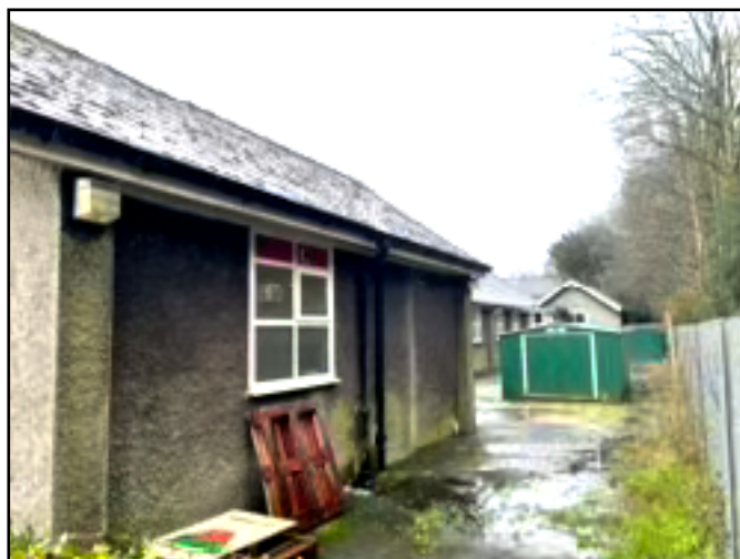
Photo 10. View along far north hardstanding area of school grounds, adjacent to railway embankment.
