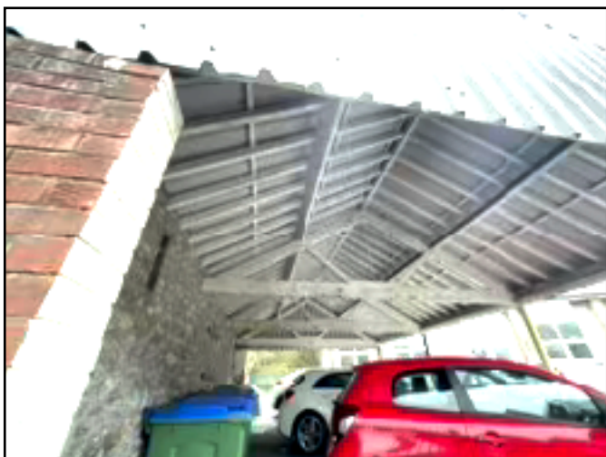
Photo 9. Car shelter structure roofing.
