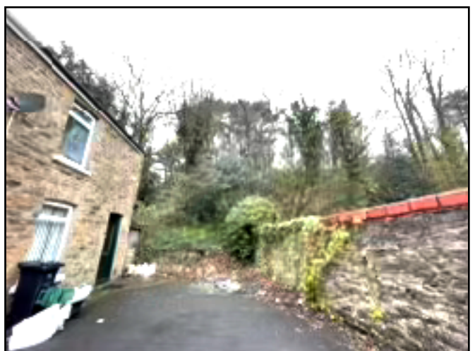
Photo 6. View of adjacent access road to west of school with northern railway embankment and stone wall creating western boundary.
