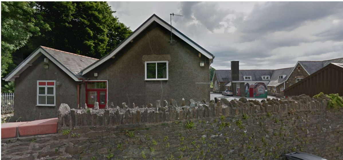
End of building facing east
