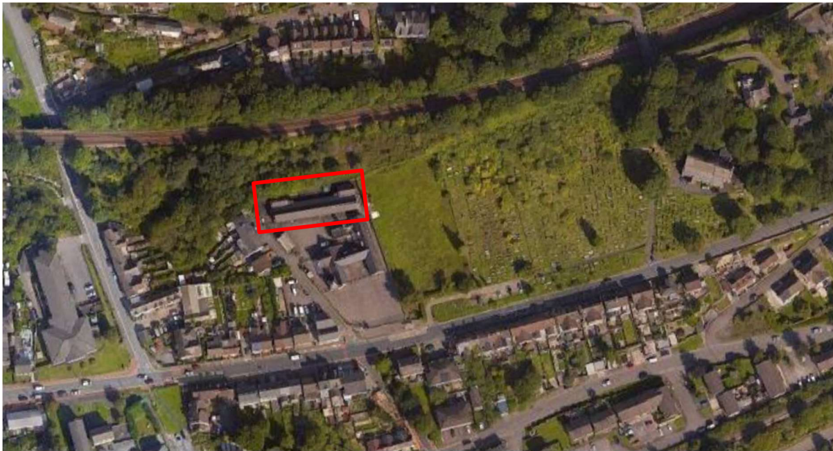
Figure 1 - Site location, block to be demolished highlighted in red
