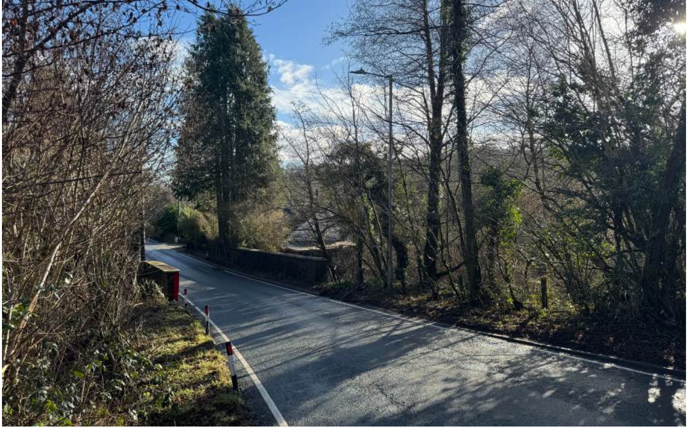
View 4 - Approaching from West - from a distance
