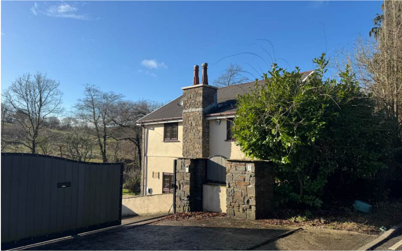
View 1 - Approaching from East - Driveway
