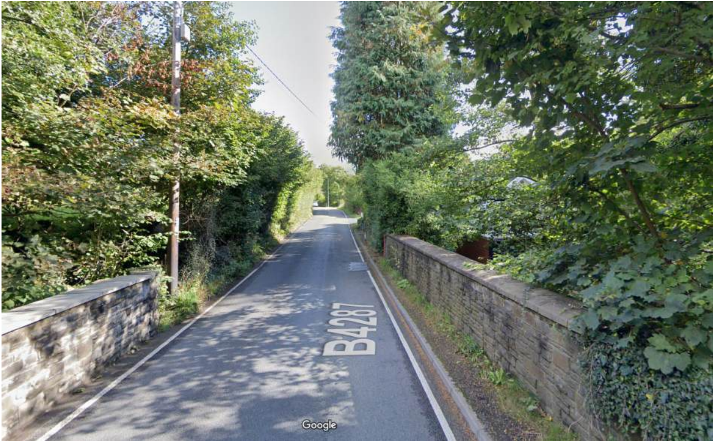
View from Lane North West (Google Street view - 2022)
