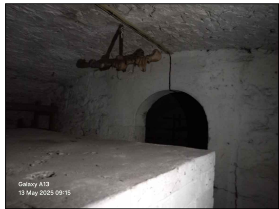
Roosting Features Surveyed
