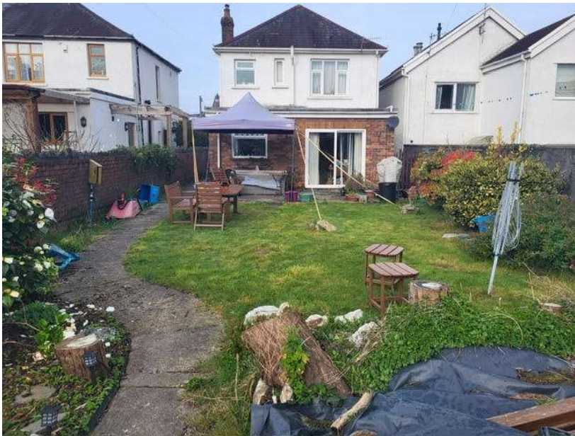
View of rear elevation and large lawned area to rear garden. Existing patio can be seen adjacent the rear elevation where the new ground floor single storey extension will be sited.
