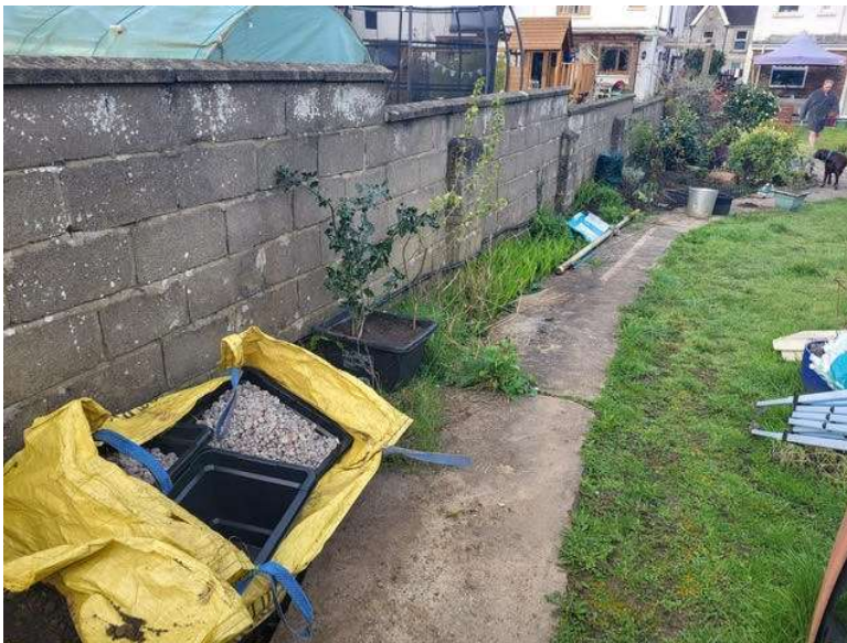
View of rear garden and neighbouring boundary to other side including blockwork boundary wall
