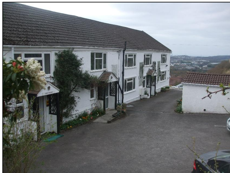
Photo 1 – View of the front elevations of the Guest House and Adjoining Dwelling
