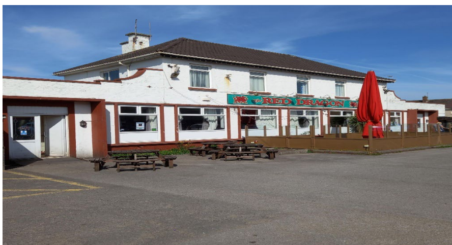
Asbestos Removal, Soft-strip and Demolition
