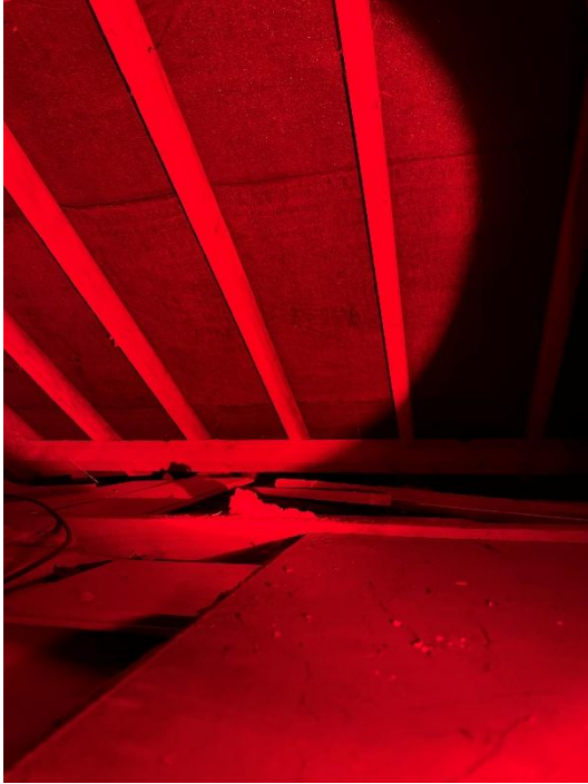
Plate 1 - Internal loft space
