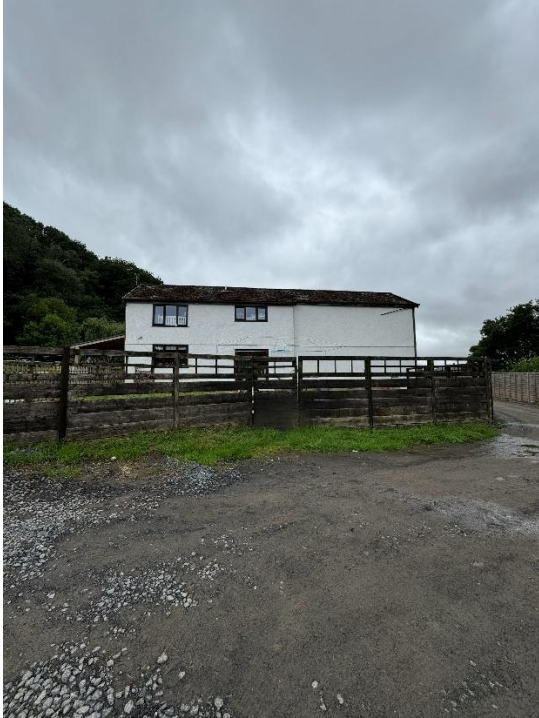
Plate 5 - Back elevation of the property
