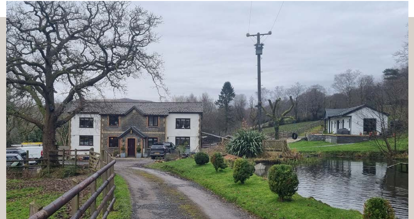
► Image 26: Existing property taken from main vehicular access approach
