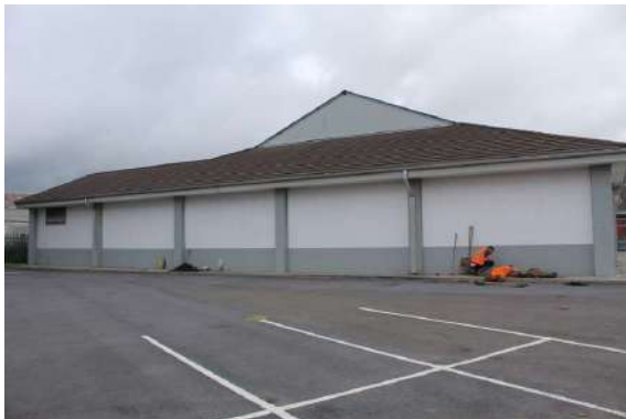
Photo 1: View northwards of the southern façade of the existing Lidl store building in July 2020.
