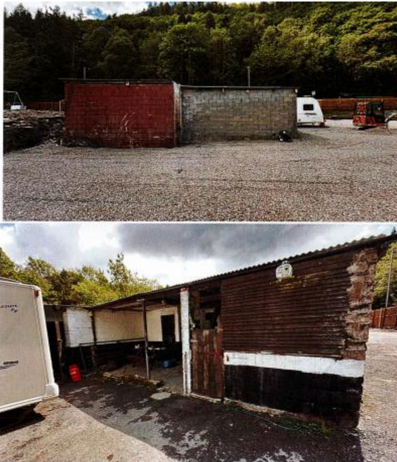
Photos showing the existing flat roof stable and storage barn proposed to be converted to two day / utility rooms
