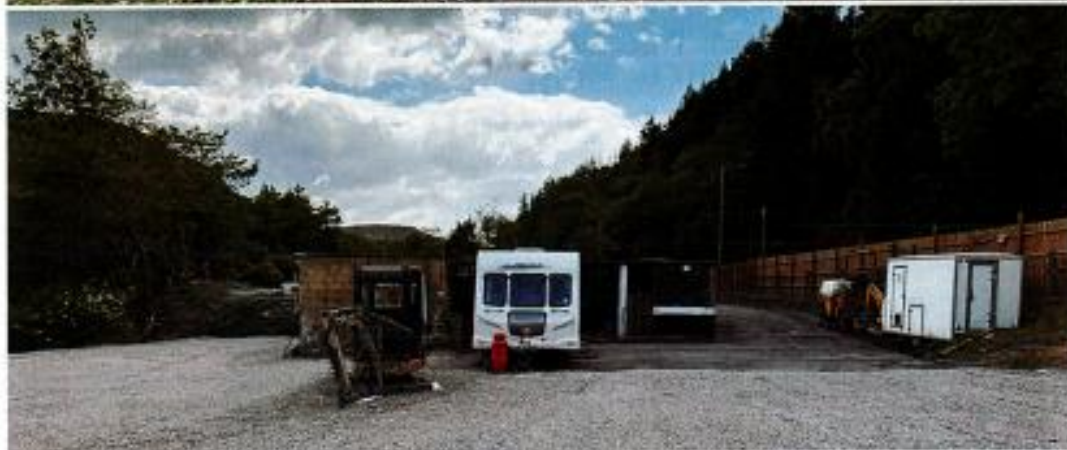
Photos of the existing site showing the levelled and rolled (crushed stone) surface
