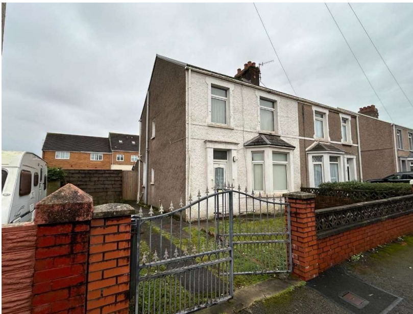
Front elevation view showing small lawn area and concrete driveway to the side of the property
