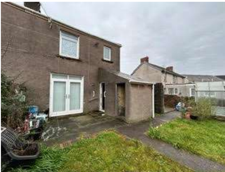
Rear elevation view including lawns, small patio area and existing lean to building to be demolished. This is the area where the rear extension will be sited.
