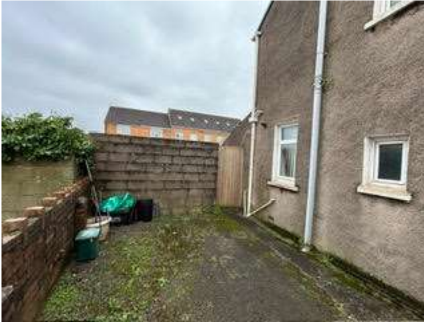
View of side elevation including concrete driveway. This is the area where the new side extension will be sited. No green space or habitats will be removed.
