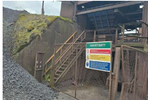
Fig.68 Conv. 731 ramp wall
