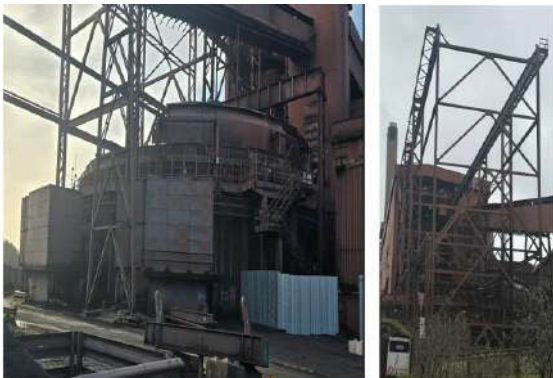
Fig.41: Sinter cooler and fan and Sinter cooler shelter.
