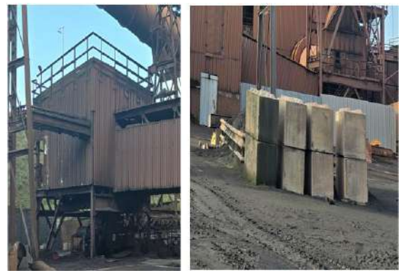
Fig.43: 1026/1027 Junction House and Lego blocks
