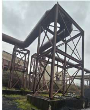
Fig.25: Junction House and Pipe Supports.
