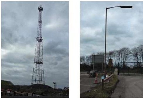
Fig.56 Light Tower and Street Light poles
