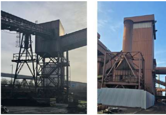
Fig.39: 1090/1091 Junction House and Mixing drum and chimney.
