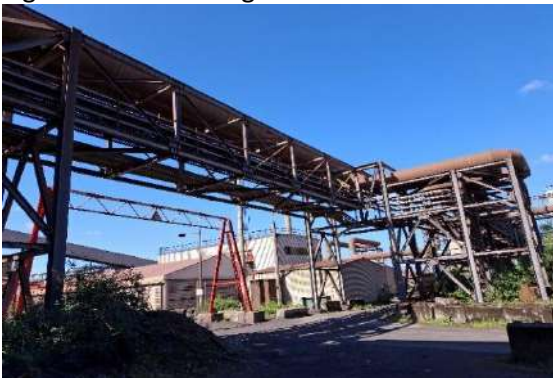
Fig.88: Pipe Works & Road Height Barrier
