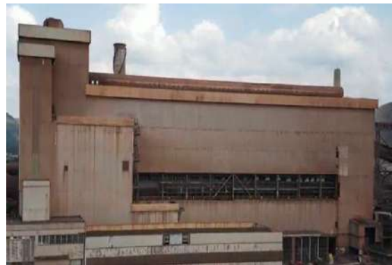
Fig 45: Sinter Plant building
