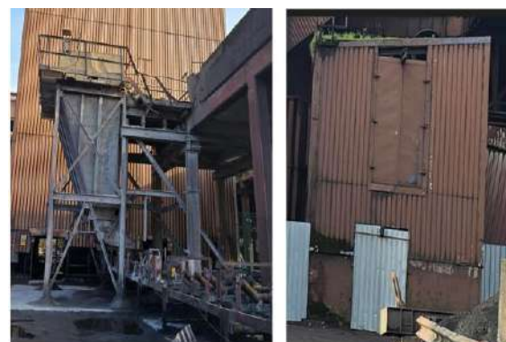
Fig.46: Limestone Bunker and 1004/1005 Junction House
