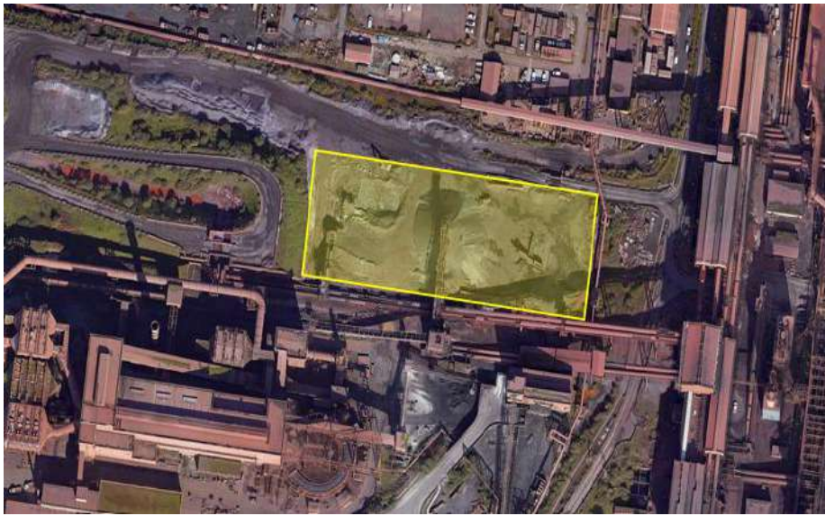
Fig 7: Lay down area (Marked in Yellow Box) – Phase G
