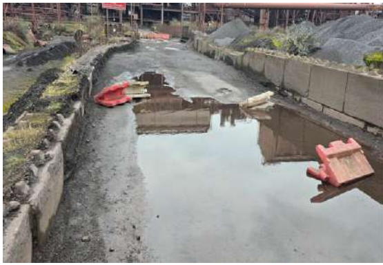
Fig.63: Lego block barrier
