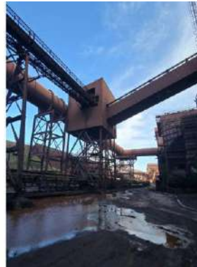
Fig.33: Fume extraction de-dusting pipe and Conv. 887/888
