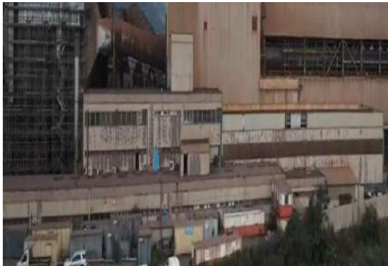
Fig.50: Sinter Building and workshop
