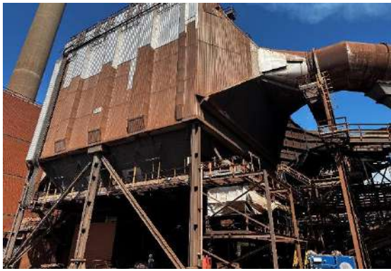
Fig. 15: Side view of Electrostatic Precipitator (3nos).
