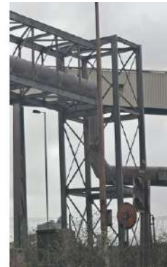
Fig.28: Conv 1082 Support Trestle and Pipe Bridge support
