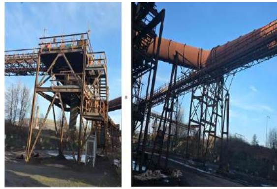
Fig. 19: Transfer House 1 for Conv 886/887 & Conv 887.
