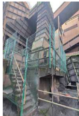
Fig.38: De-dusting precipitator fan motor support and De-dusting precipitator duct to stack and inlet plenum.
