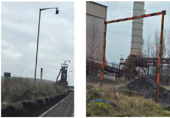
Fig.79: Light Poles and Truck Barrier
