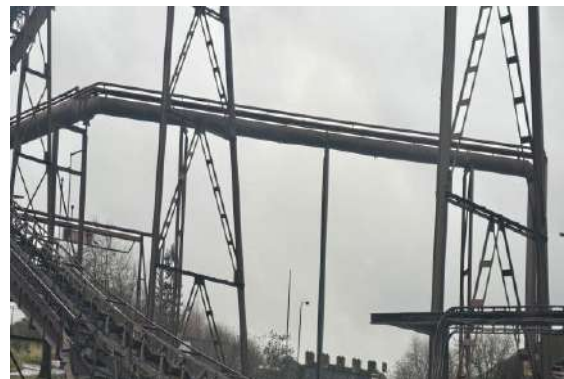
Fig.30: 800mm Dia Pipe & Trestles
