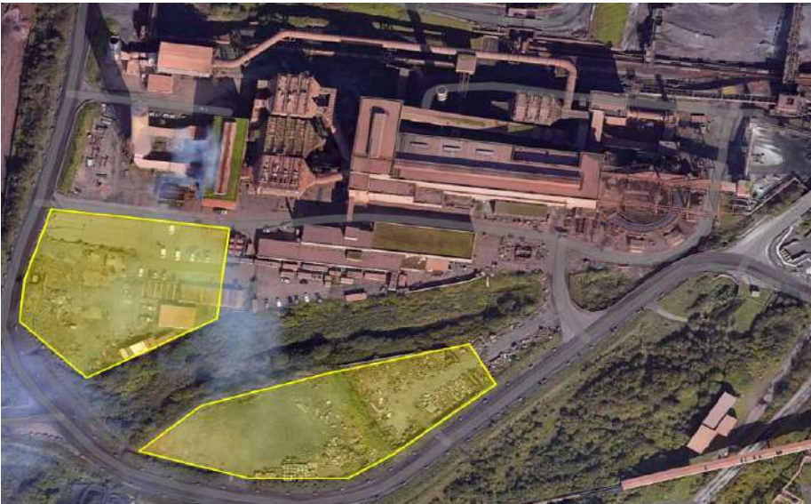
Fig 5: Lay down area (Marked in Yellow Box) – Phase D & E
