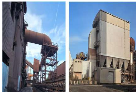
Fig. 14: Fume extraction ducting and De-Dusting Building
