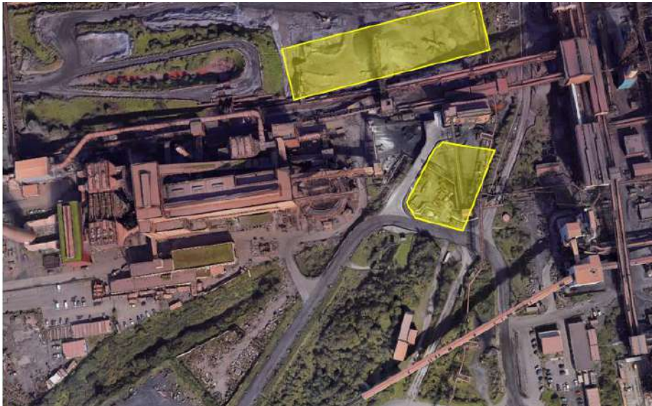
Fig 4: Lay down area (Marked in Yellow Box) – Phase C
