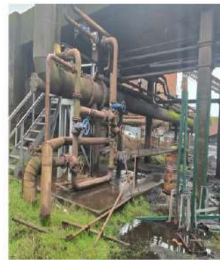
Fig.27: Conv 1080 and Sinter Plant Water Systems-Rod Mill Water
