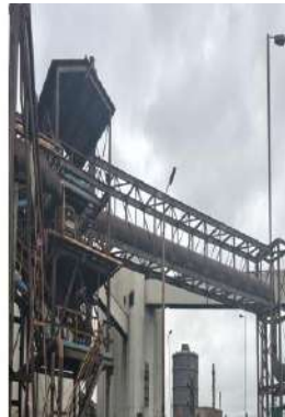
Fig.24: Spillage Bay and Pipe Bridge.
