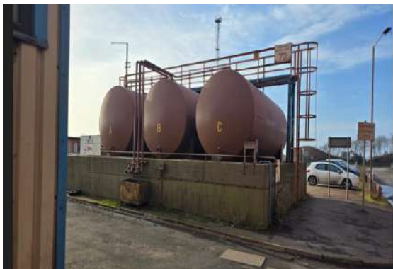
Fig 51 : Heating Tanks
