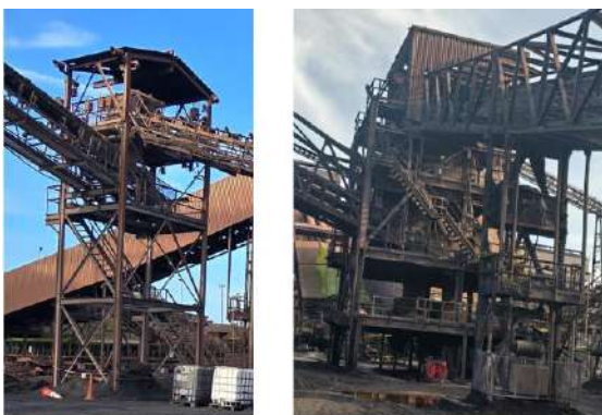
Fig.42: 1089/1090 Junction House and 1027/1028 Junction House.
