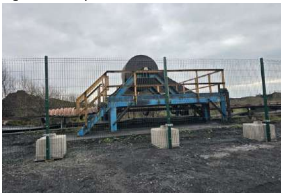
Fig.58: Conveyor 1402 Head Drum
