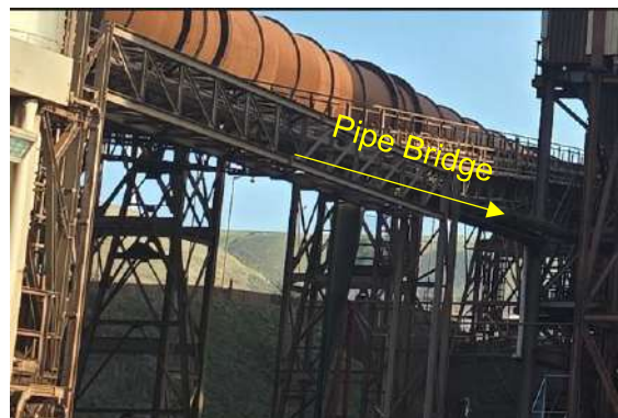
Fig. 21: Pipe Bridge.
