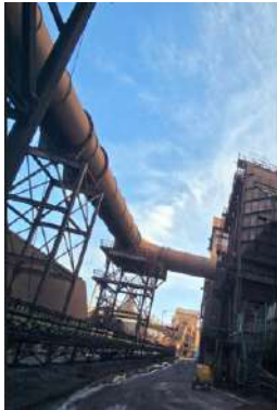
Fig.33: Fume extraction de-dusting pipe and Conv. 887/888
