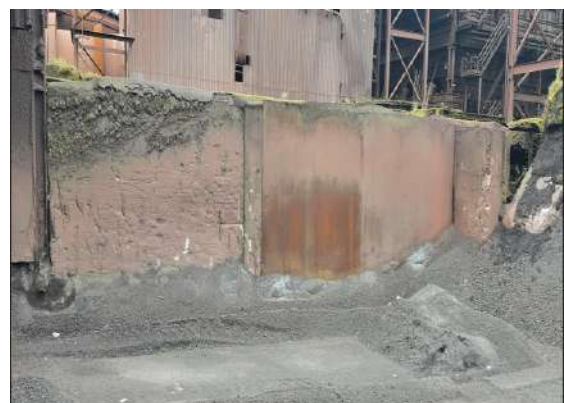
Fig.70 Junction house 731/735 retaining wall
