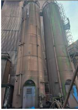
Fig.31: Coke and Lime Silo and De-Dusting Precipitator Stack (Chimney)
