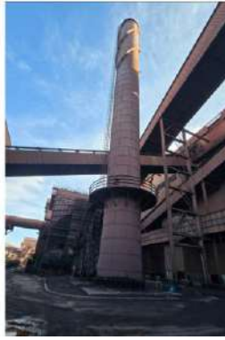
Fig.31: Coke and Lime Silo and De-Dusting Precipitator Stack (Chimney)
