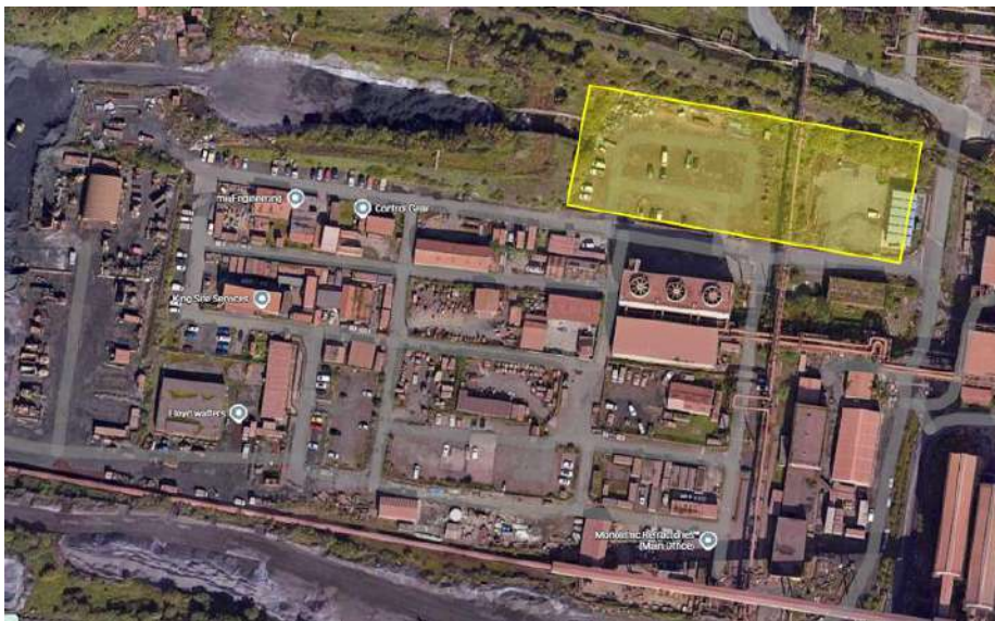
Fig 8: Lay down area (Marked in Yellow Box) – Phase H
