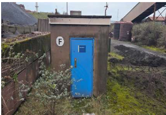
Fig.65 Wheel wash control building
