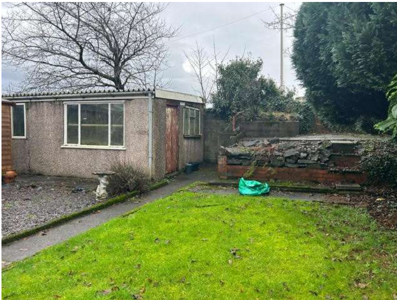
View of rear boundary including existing detached garage, blockwork boundary wall and mature trees which are all to remain. Large lawn in foreground.
