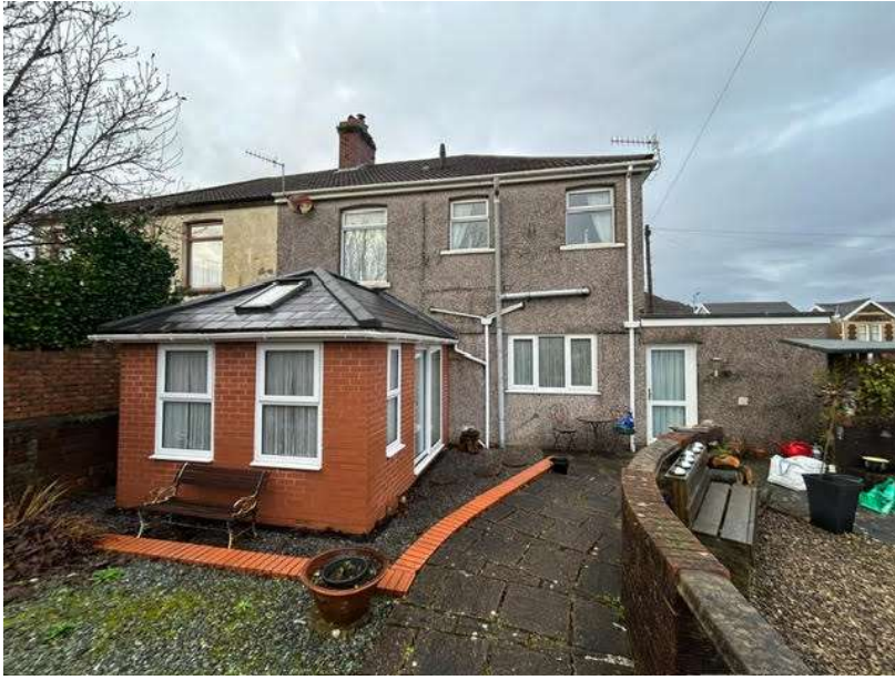
Closer view of rear elevation where new extension will be sited
