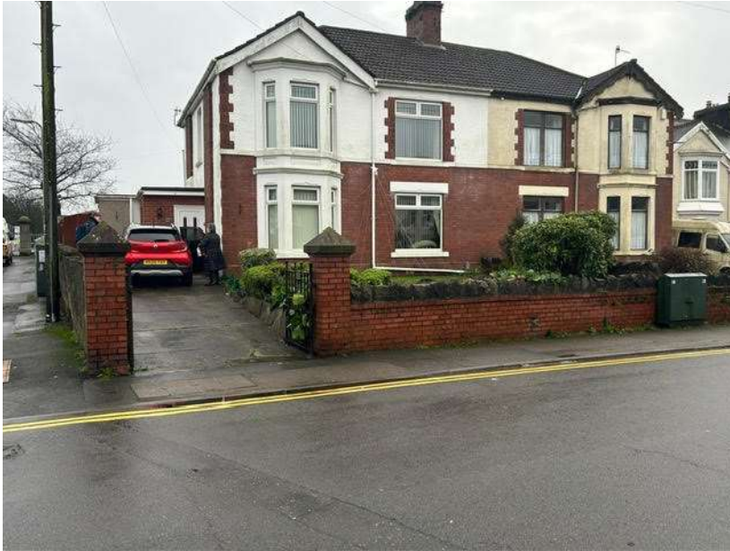
View of front elevation including brickwork boundary wall with concrete driveway and lawned area with planted borders.
