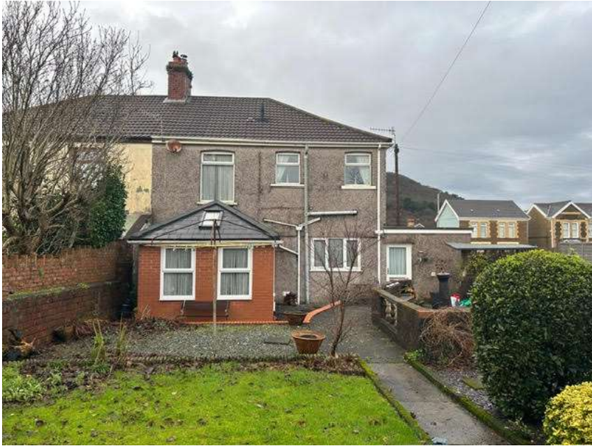
View of rear elevation showing area where single storey and two storey extension will be sited. No green space or habitats will be removed. The extension will be sited where there is a current extension or onto patio area.
