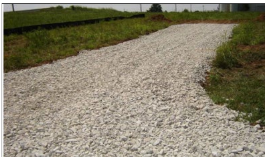
Figure 2: Temporary access track
