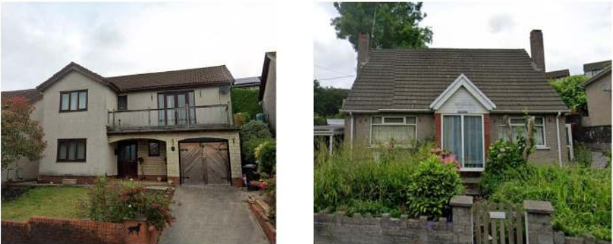
Dwellings along Cardonnel Road showing the variety of forms/styles
