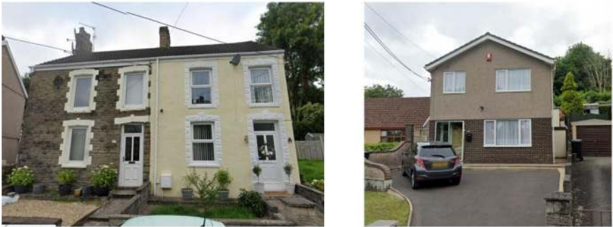
Dwellings along Cardonnel Road showing the variety of forms/styles
