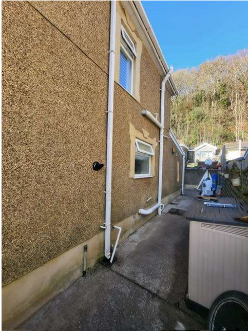
Side elevation view including concrete path leading to the rear garden areas.
