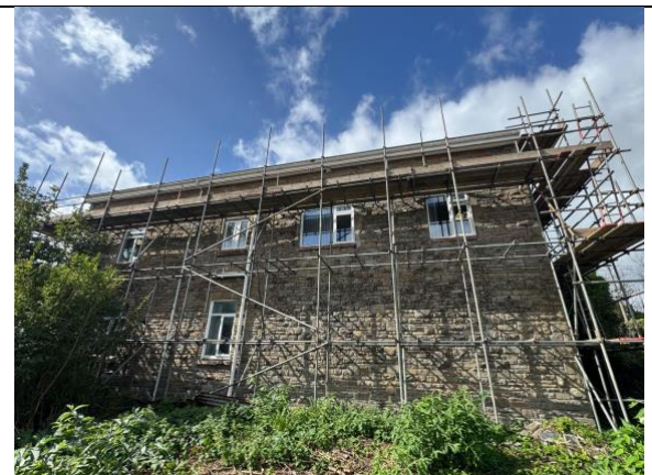
Rear southeast facing aspect of the property
