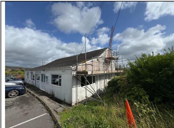
Side southwest facing aspect of the property
