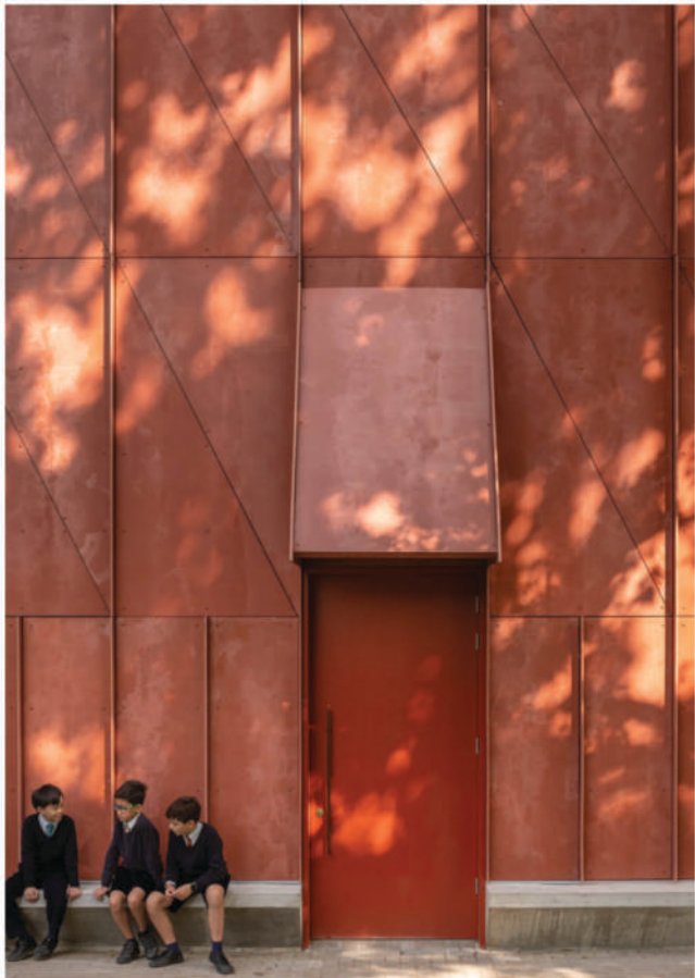
Viroc panels and concrete plinth
