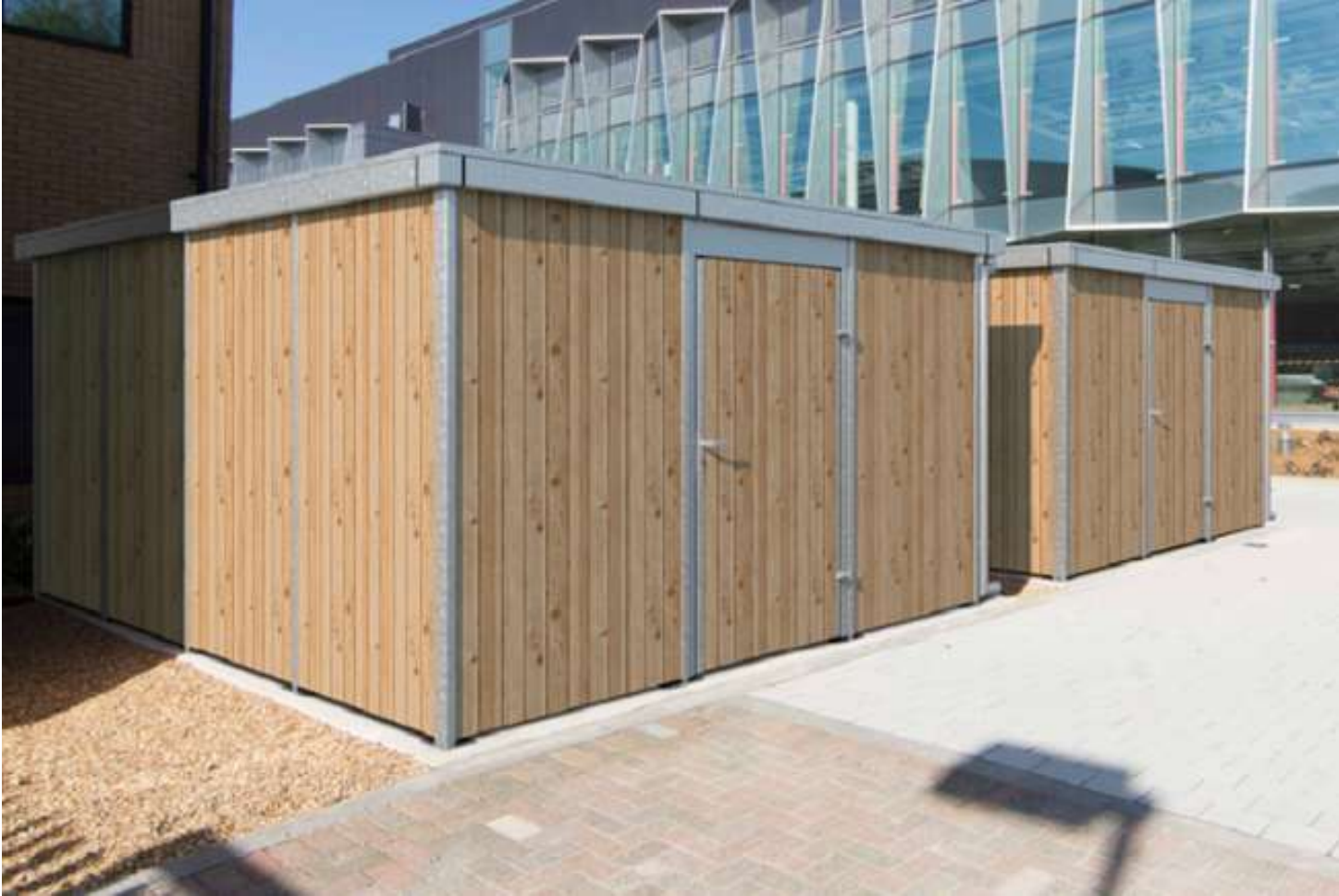
Bin Store Enclosure
