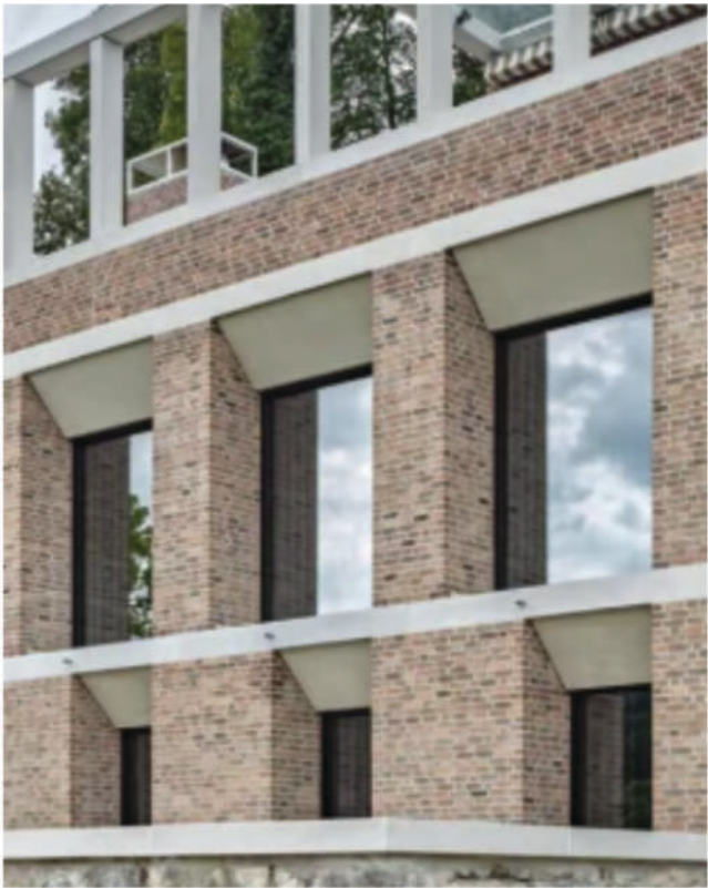
Window reveals with chamfered head
