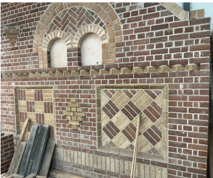
Bricklaying wall exemplar
