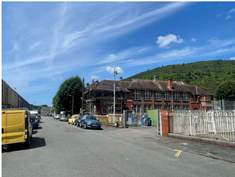
1. View from the east side of Reginald Street
