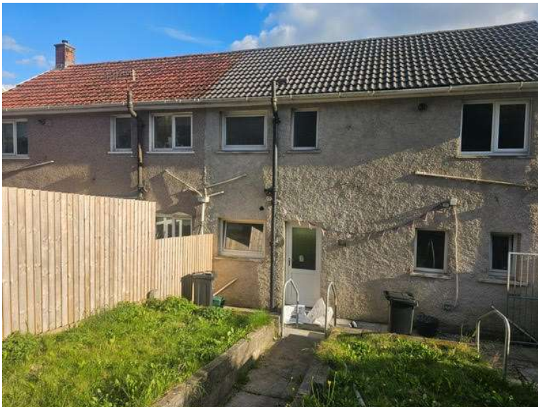
Rear elevation view showing small patio area adjacent rear elevation, timber fence boundary and lawn areas.
