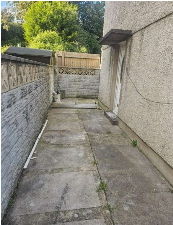
Side elevation view of concrete path to rear garden area and front door
