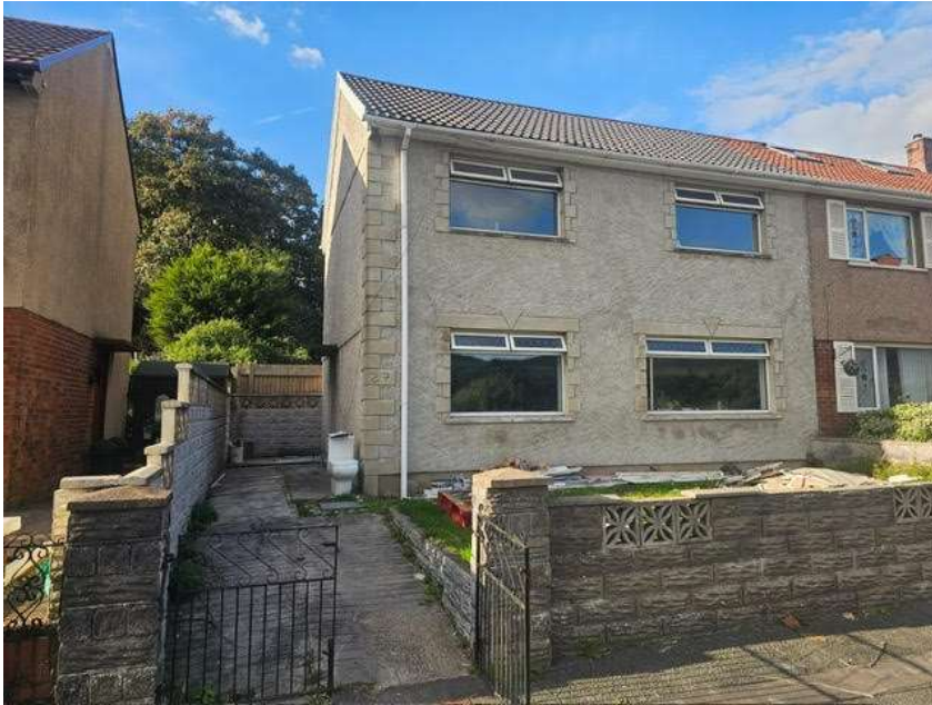
Front elevation showing concrete path and small lawn area.
