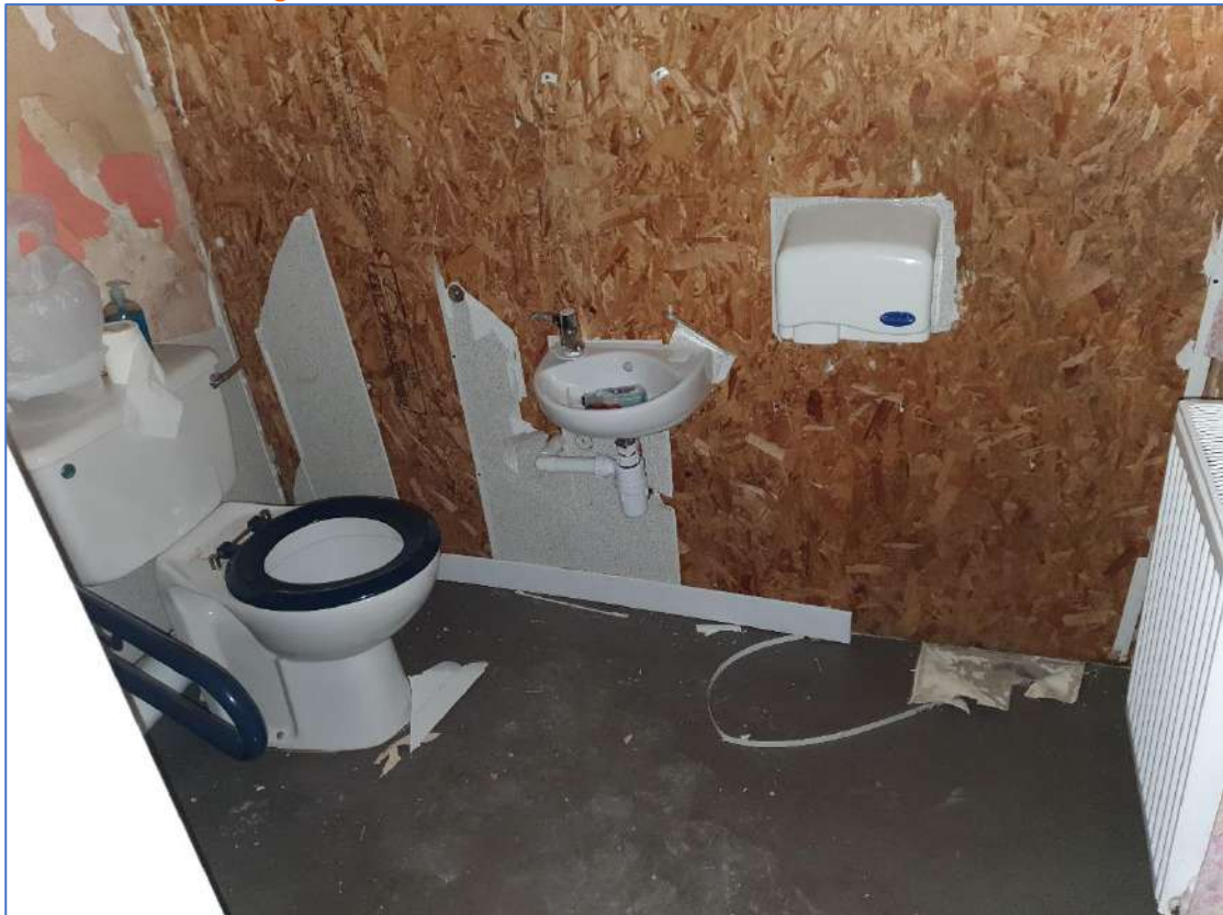
Photo 6 – Toilet on the ground floor
