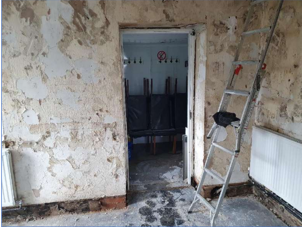
Internal Doorway (Bar)
