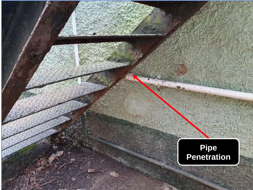
Pipe Penetration – North Western Perimeter
