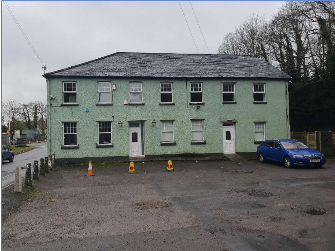
Photo 1 – North eastern perimeter of the property
