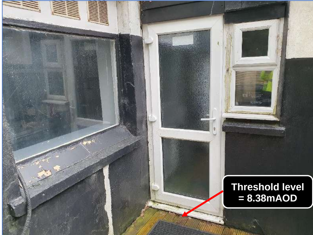
Single Door – North Western Perimeter
