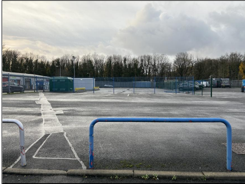
Photograph 4 – The Site Looking West
