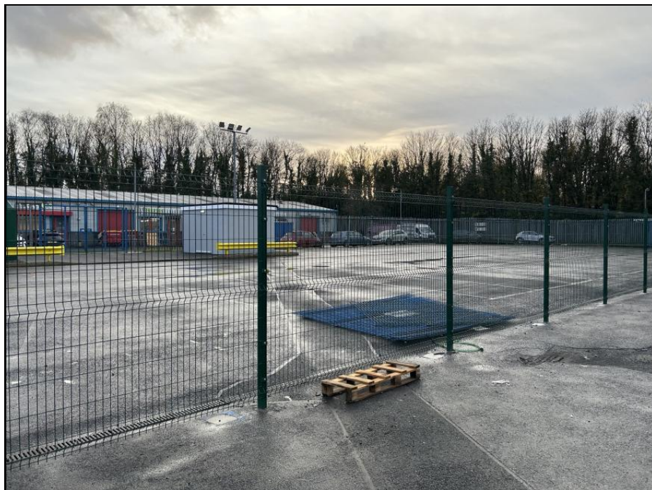
Photograph 5 – The Site Looking Southwest from Toolstation Car Park
