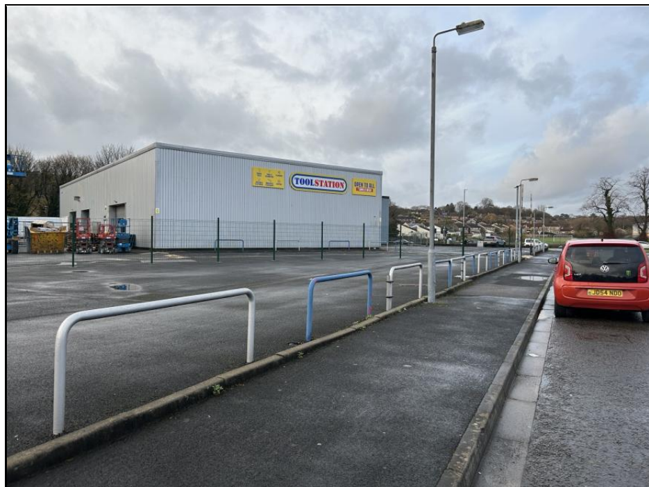
Photograph 3 – The Site Looking North with Toolstation Visible
