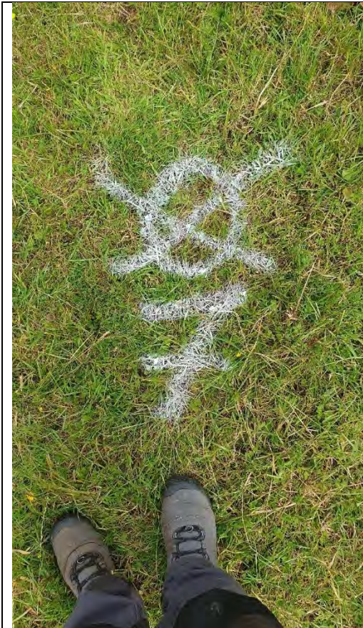
PSP07 – Borehole location
