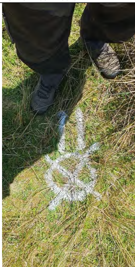
PSP11 – Borehole location
