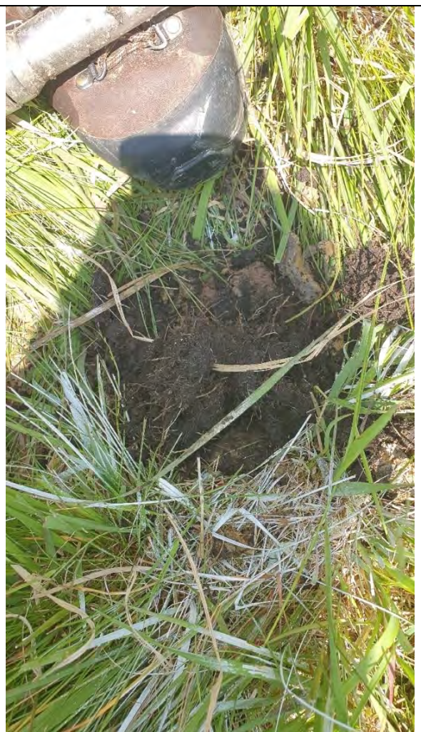
PSP17 – Borehole reinstated
