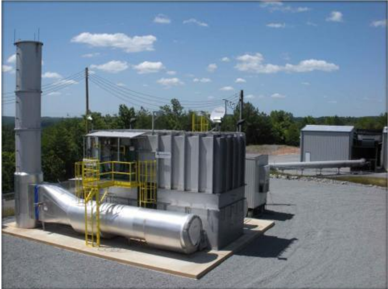
Typical VAM Oxidizer Setup.
