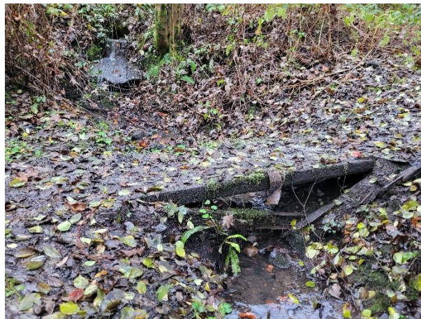
Photo 8: Existing Watercourse Crossing
