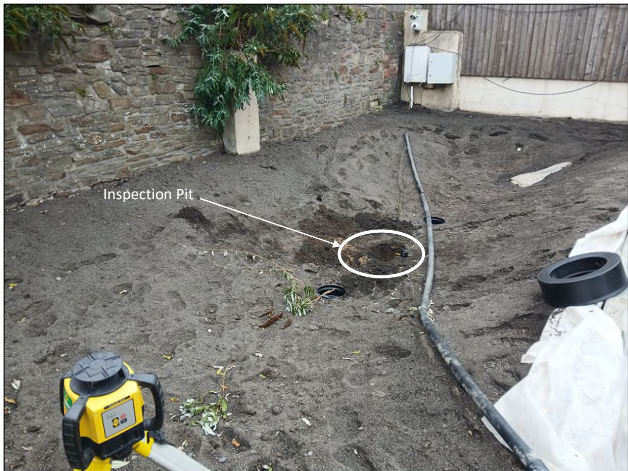
Figure 3.2: Inspection Pit Location Within SuDS Basin
