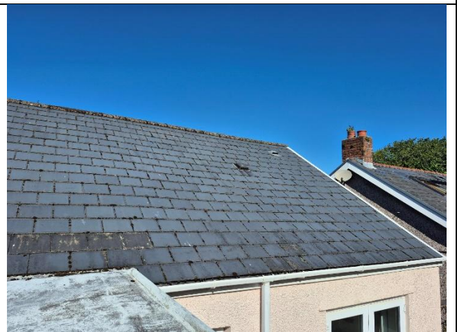
Photo 3. Roof of the Property
