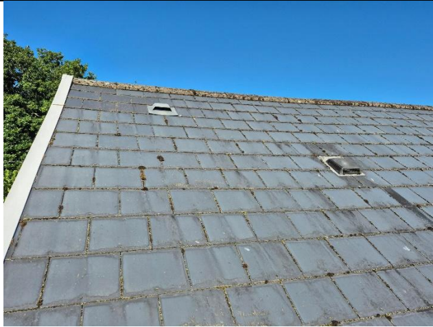
Photo 4. Roof of the Property
