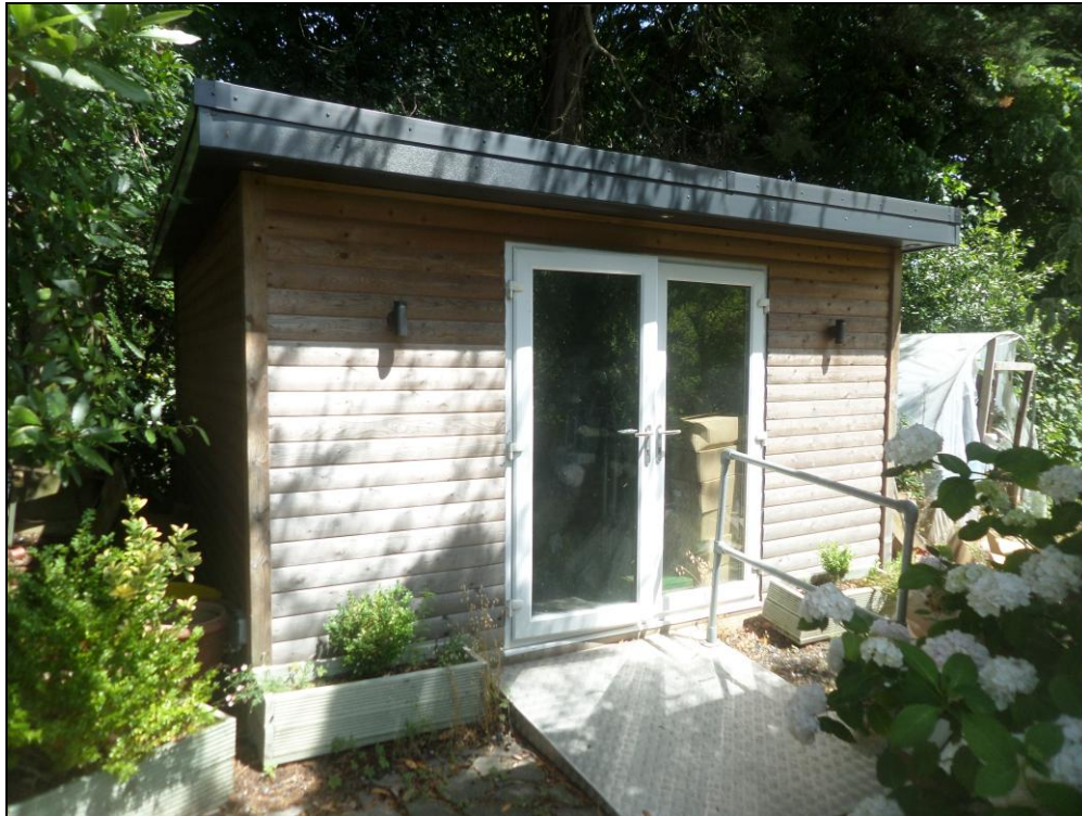
Photo 15: Northern storage building (view looking south west).
