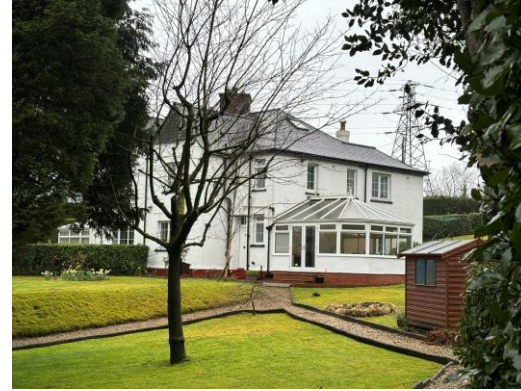
FIG 32 VIEW OF No 18 CEFN-PARC ROAD
