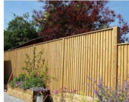
FIG 75 – ILLUSTRATIVE EXAMPLE CLOSEBOARD FENCE
