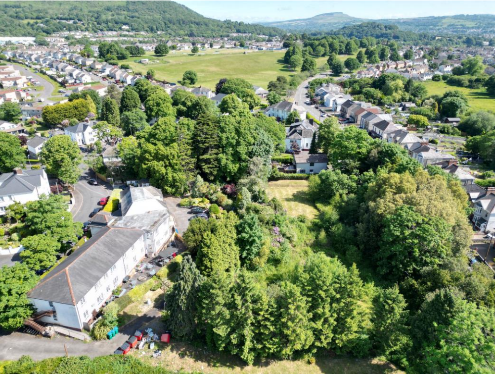
FIG 31 – SITE VIEW FROM SOUTH
