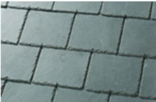
NATURAL SLATE ROOF
