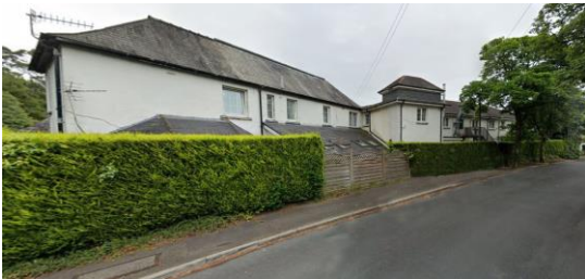
FIG 24 VIEW OF CEFN-PARC ROAD- EXISTING CARE HOME
