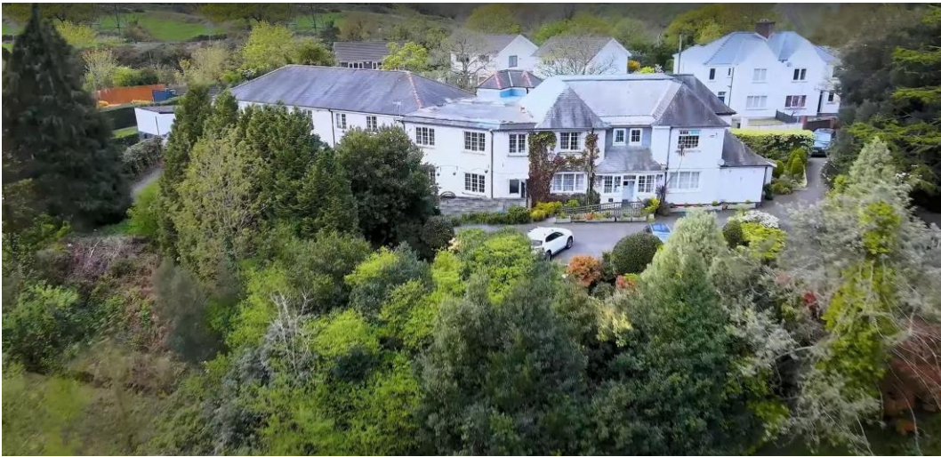
FIG 29 VIEW FROM EAST OF CEFN-PARC ROAD- EXISTING CARE HOME
