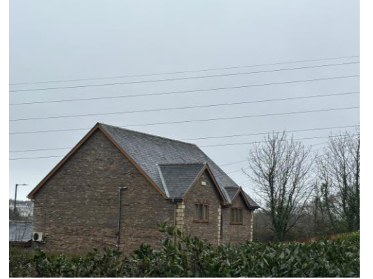
FIG 33 VIEW OF No 24 CEFN-PARC ROAD
