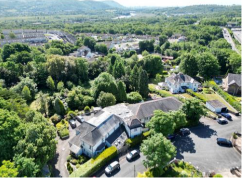
FIG 49 - AERIAL VIEW- WEST
