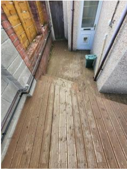
View of area where the extension will be sited over a decked area and where existing small rear porch is currently
