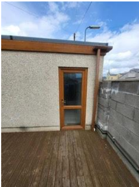
View of existing rear outbuilding with decking area
