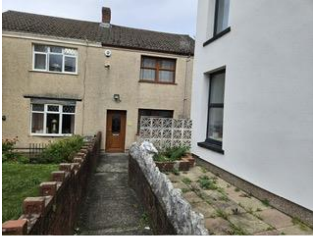
View of front elevation with concrete path to front entrance door
