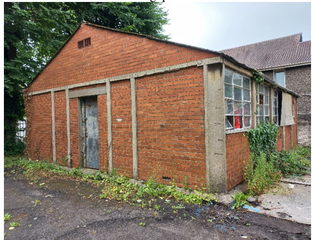
B2, found in the south-western corner of the site
