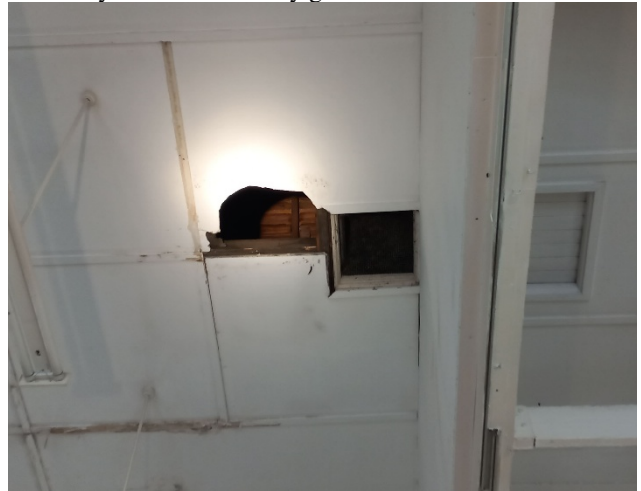
View into B1 loft void from gap
