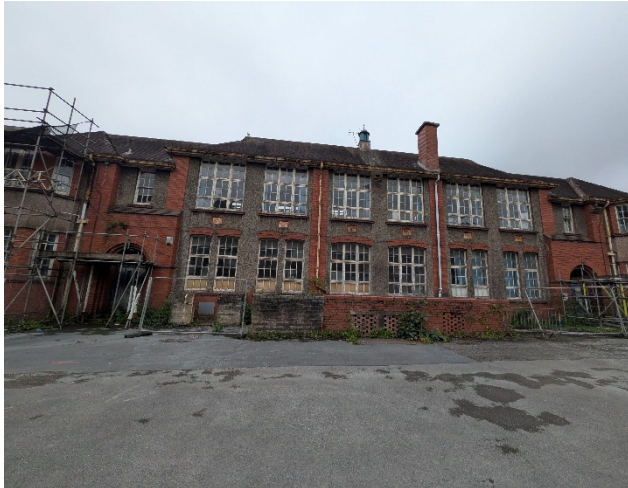
B1 exterior and entrance, eastern elevation
