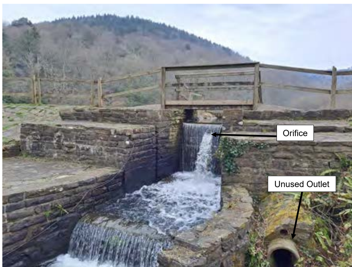
Figure 3-3 Downstream Face of Margam Duck Pond Outlet at Foot Bridge_03
