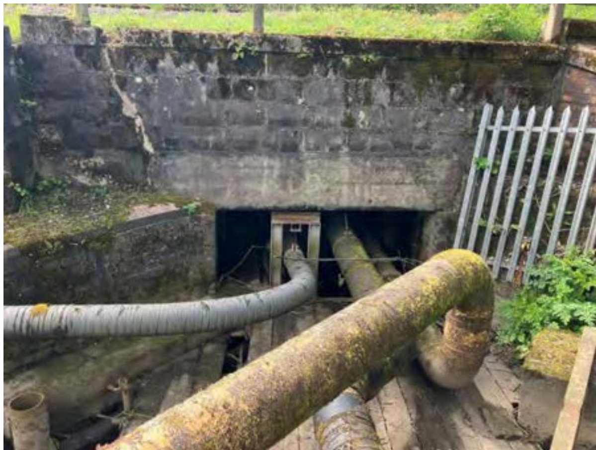
Figure 3-5: Upstream Face of TATA Steel Inlet
