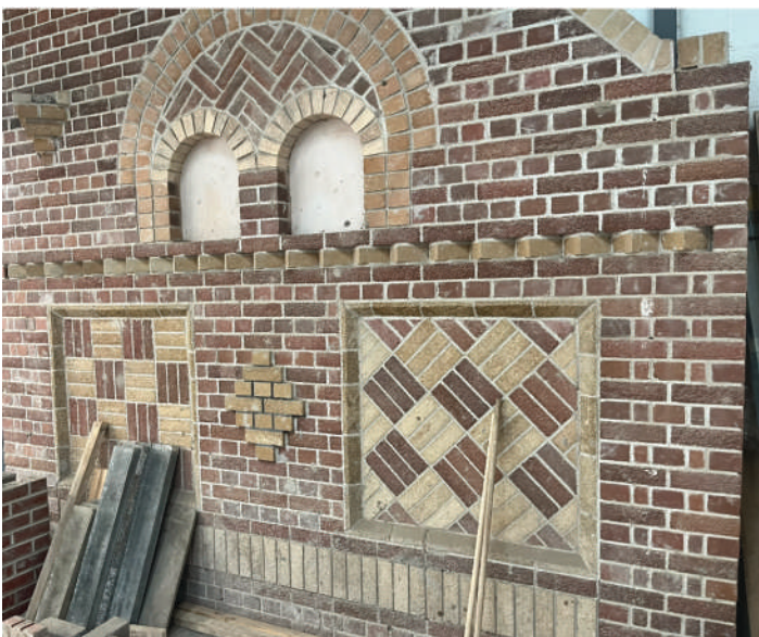
Bricklaying wall exemplar
