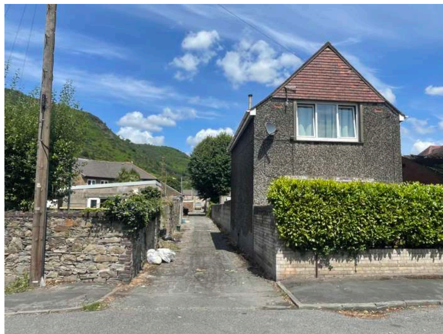
4. View of service road and old Ground keeper's house from Reginald Street
