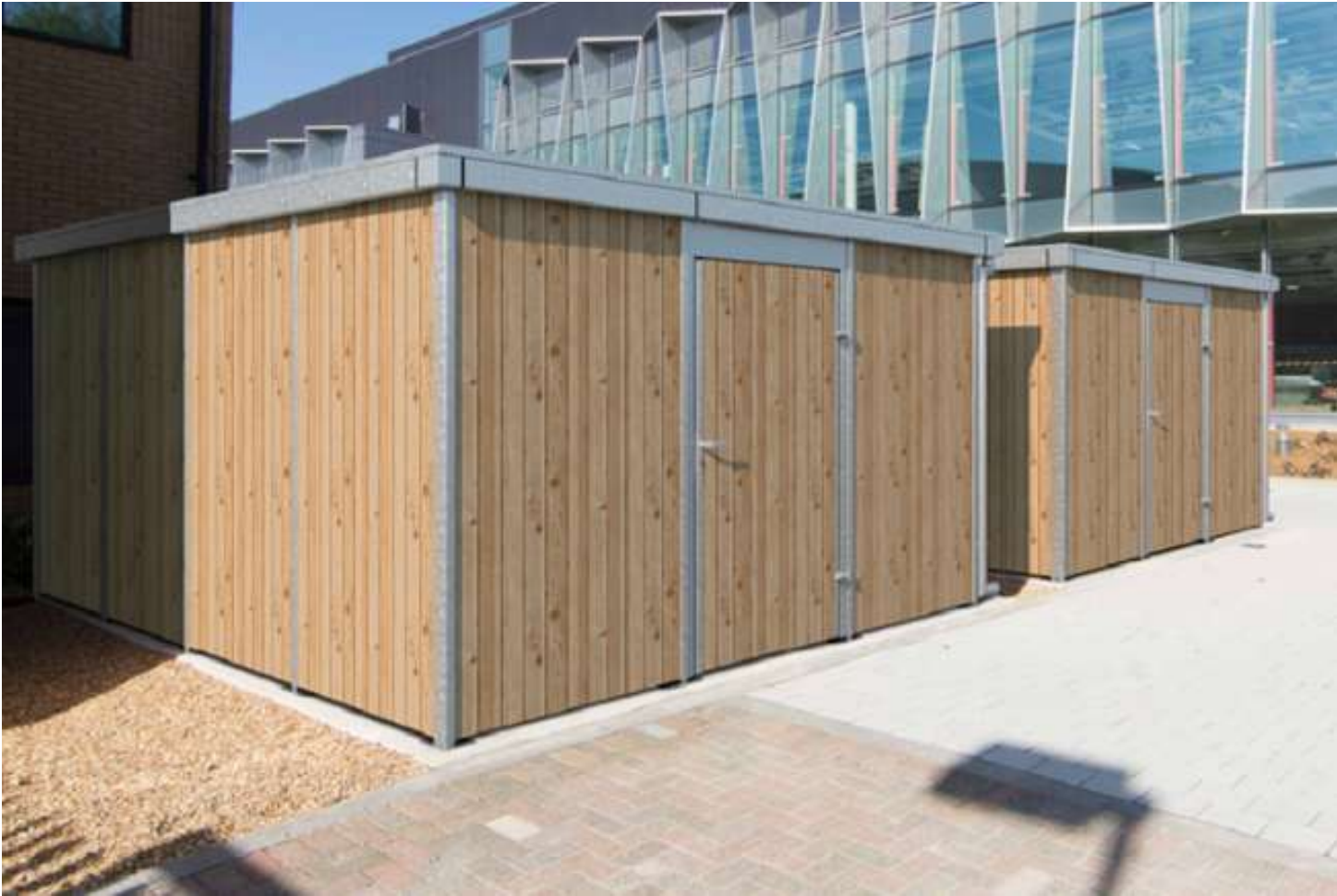
Bin Store Enclosure
