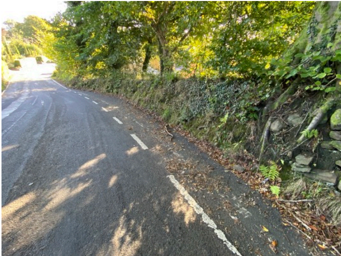
Pen yr Alltwen road viewing east, site northern boundary stone wall to the right
