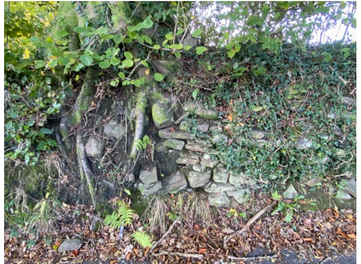
Pen yr Alltwen road site northern boundary stone wall
