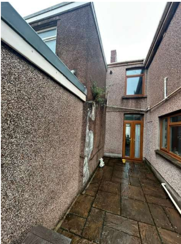
View of existing patio area where infill extension will be positioned. Neighbours existing two storey and single storey extensions can be seen.
