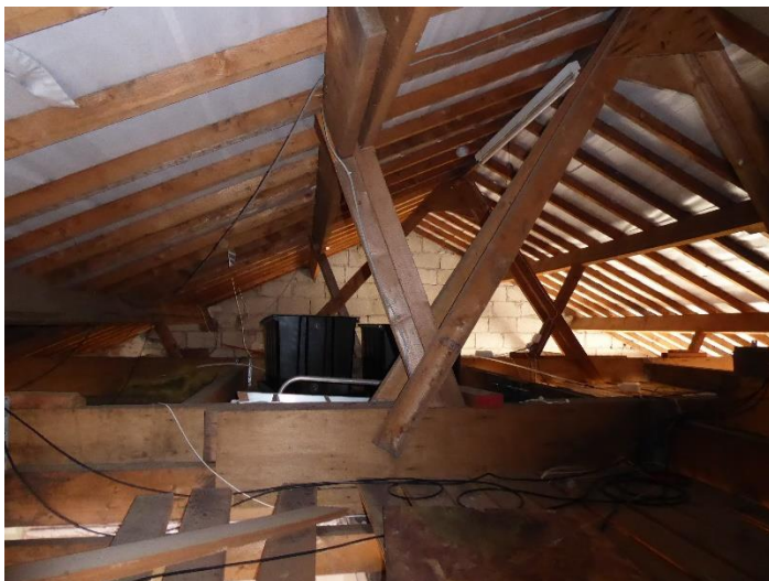
Figure 11 Existing roof loft space
