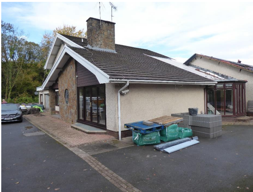
Figure 5 East elevation of property
