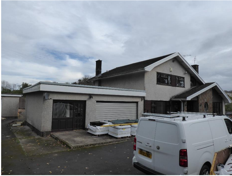
Figure 4 South elevation showing garage flat roof
