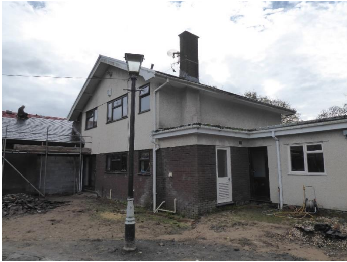
Figure 6 North elevation of property
