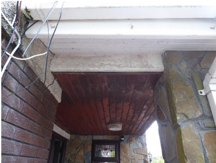
Figure 10 Front entrance canopy well sealed ceiling
