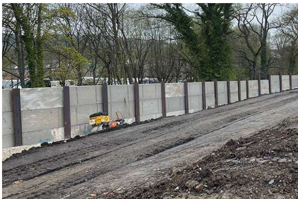
Photo: Typical kingpost wall (Credit – Craven Concrete)
