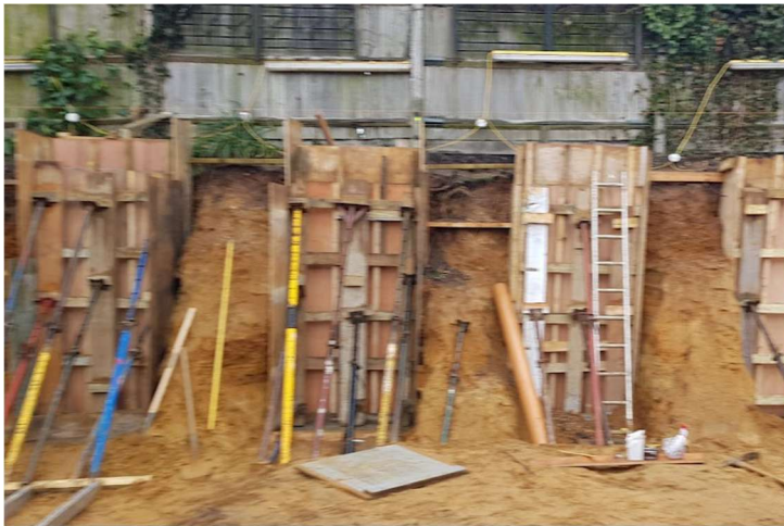
Photo: Typical sequential dig
