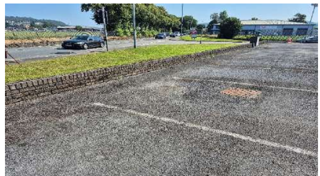
Photograph 7 – Wall and Hard Standing
