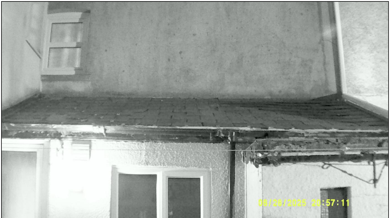
Figure 2: IR Camera view of southern extension slate roof (view looking east).
