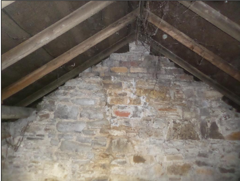
Photo 6: Exposed wooden rafters and bitumastic roof felting evident throughout (view looking west).
