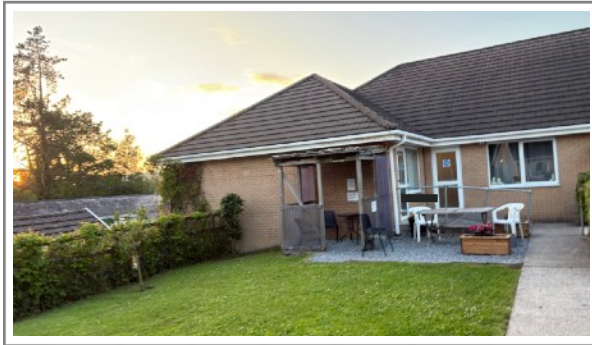
Photo 1: South facing elevations
