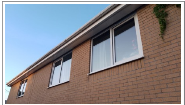
Photo 4: West facing elevations
