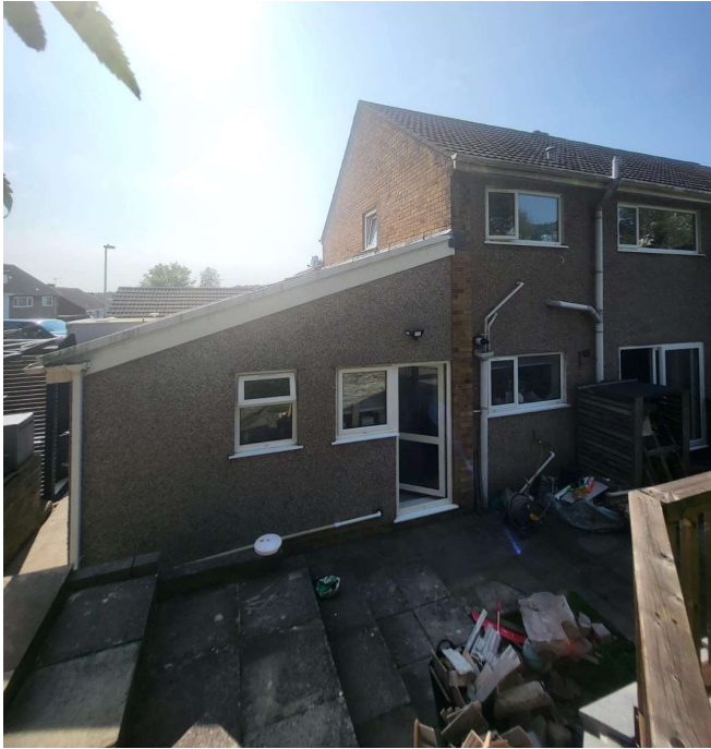
View of rear elevation and existing ground floor extension onto which the proposed extension will be sited. Existing patio also shown.
