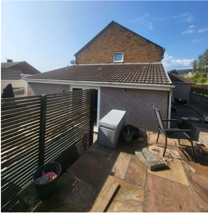
View of side elevation including enclosed patio areas and existing ground floor extension onto which the new first floor extension will be sited
