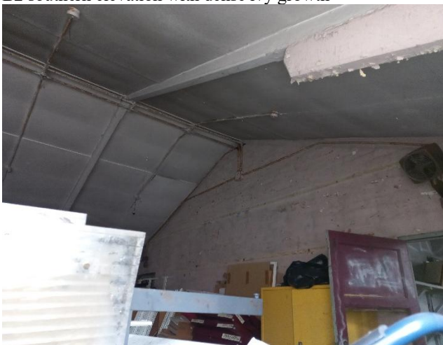
Interior of B2
