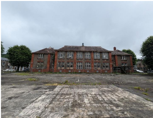
B1 exterior, western elevation
