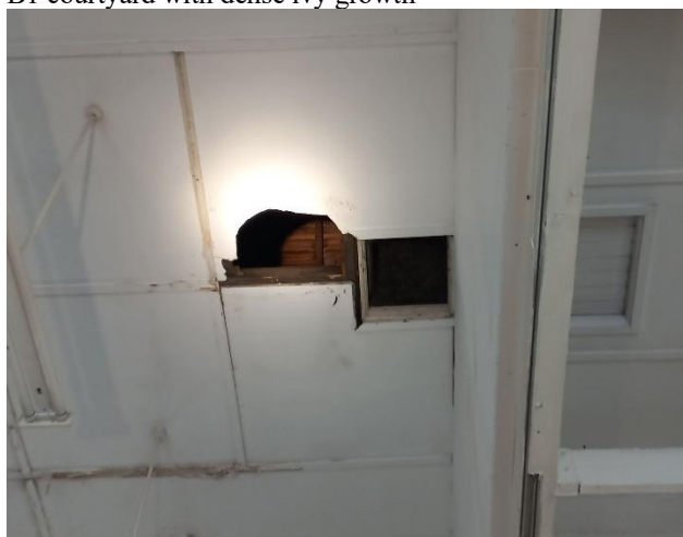
View into B1 loft void from gap
