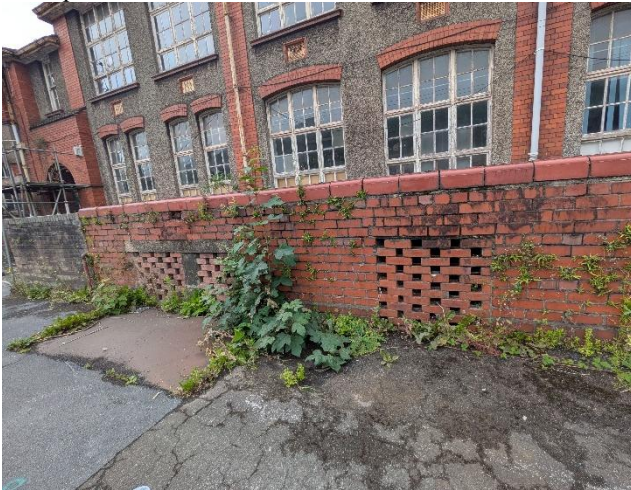
Exterior of subterranean boiler room
