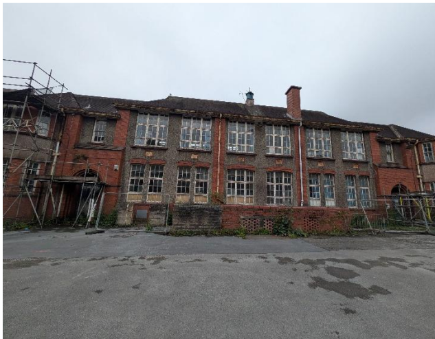
B1 exterior and entrance, eastern elevation
