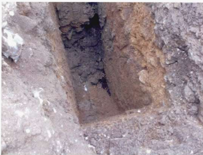
Figure 4. Free phase hydrocarbons entering the excavation from the base
