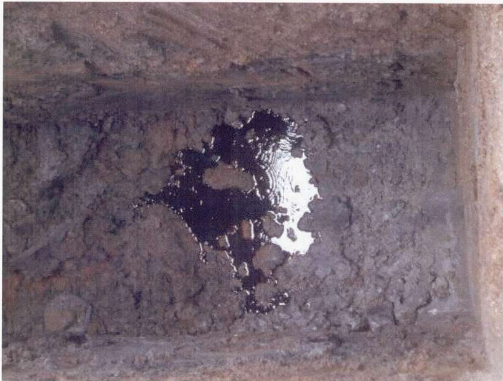
Photo 3 – Ingress of free phase product into LEE pit 7.
