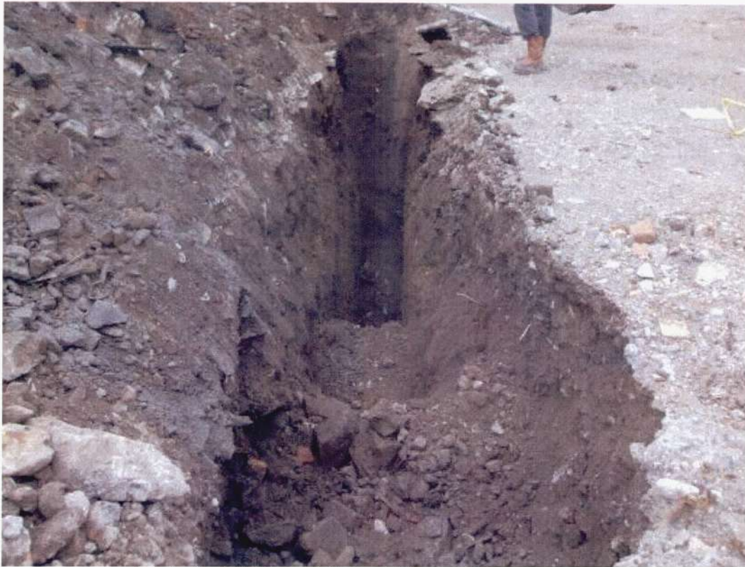
Photo 1 – Trial trench through former compound area.
