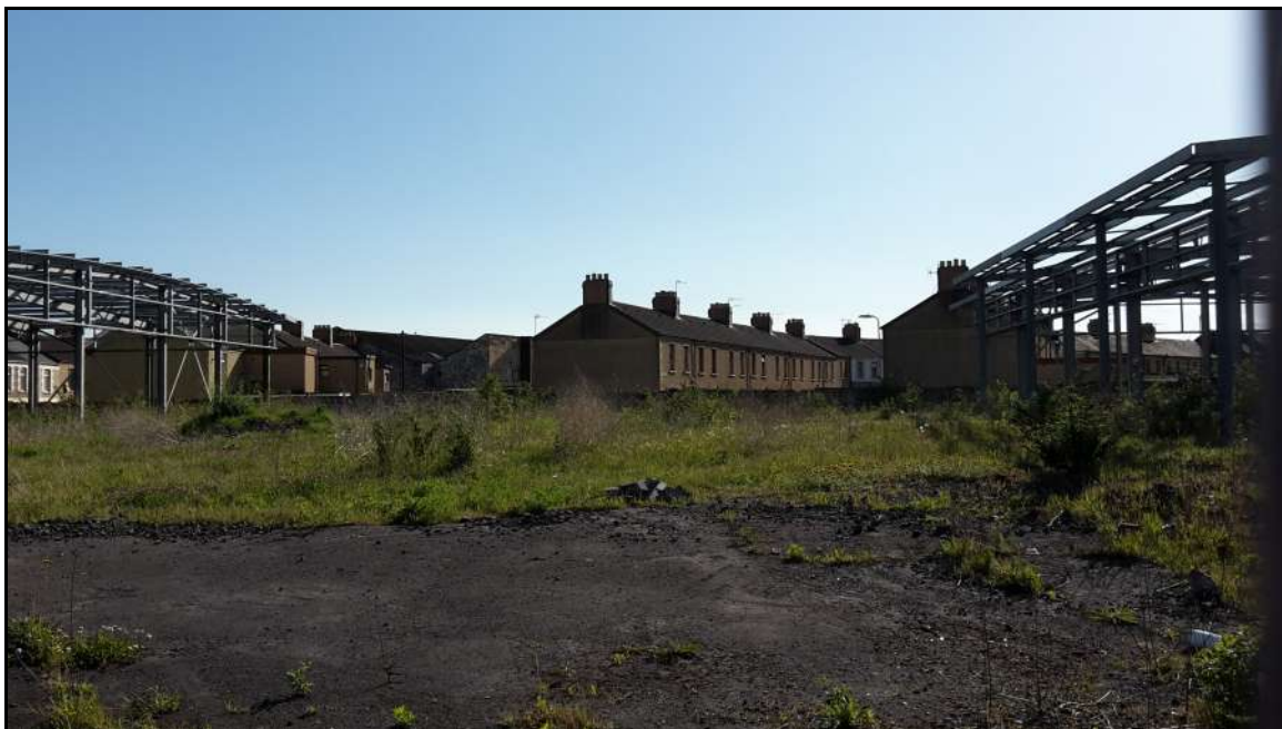
Plate 5: Area between structures, from gate.
