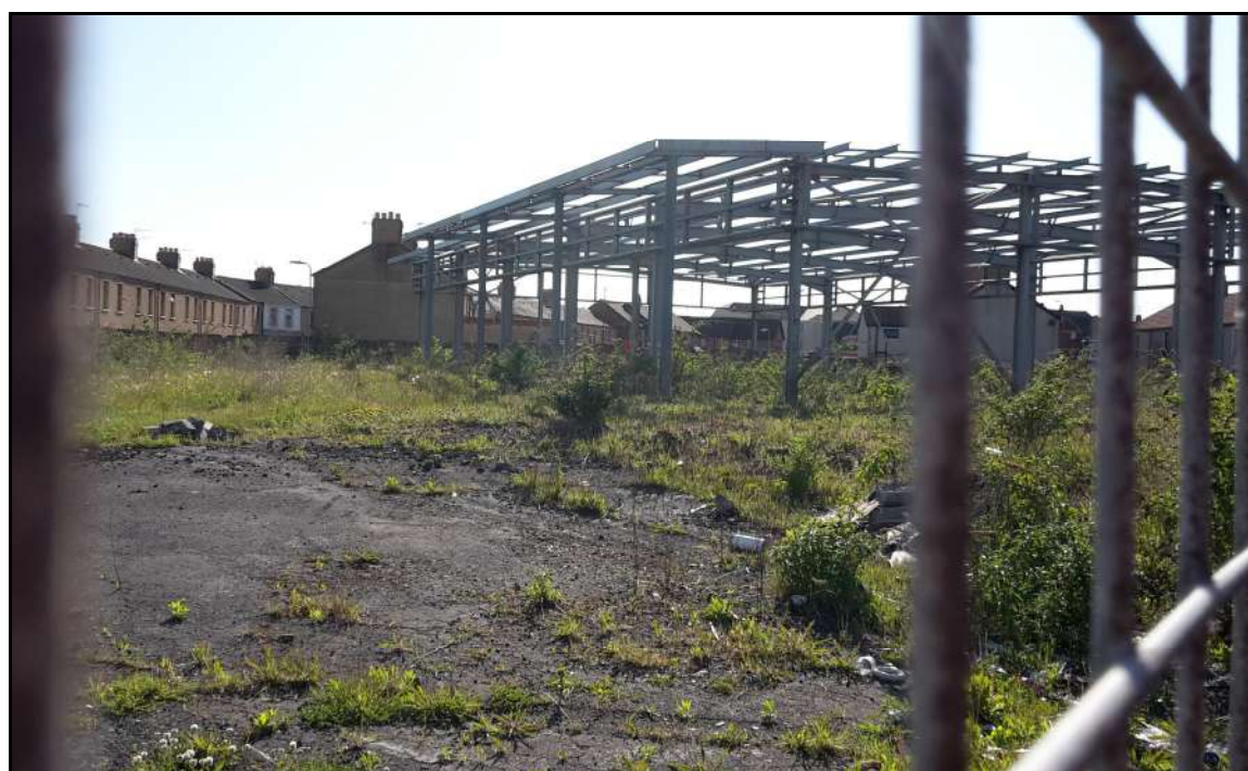
Plate 6: Northern structure, from gate.
